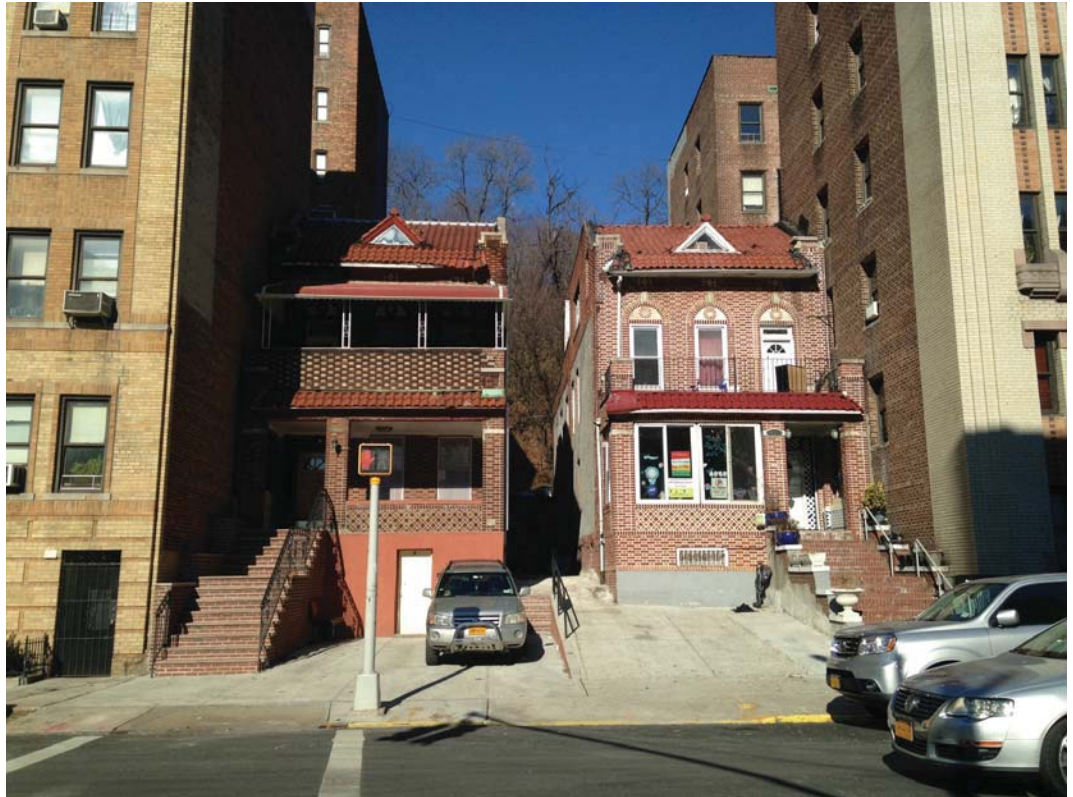
View of the project site from Seaman Avenue.
