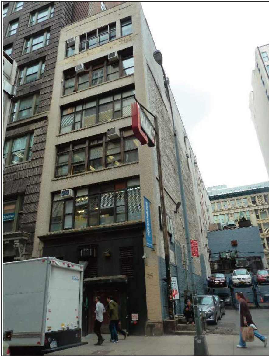
(1) West 17th Street facade of Lot 14 (42 West 18th Street/45 West 17th Street) and adjacent parking lot on Lot 15.
