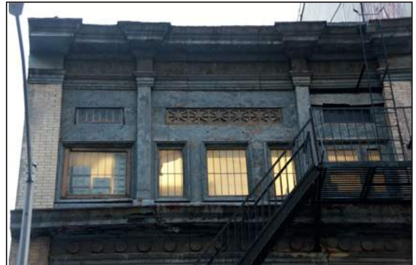
(5) Detail of upper cornice of Lot 14 on West 18th Street.
