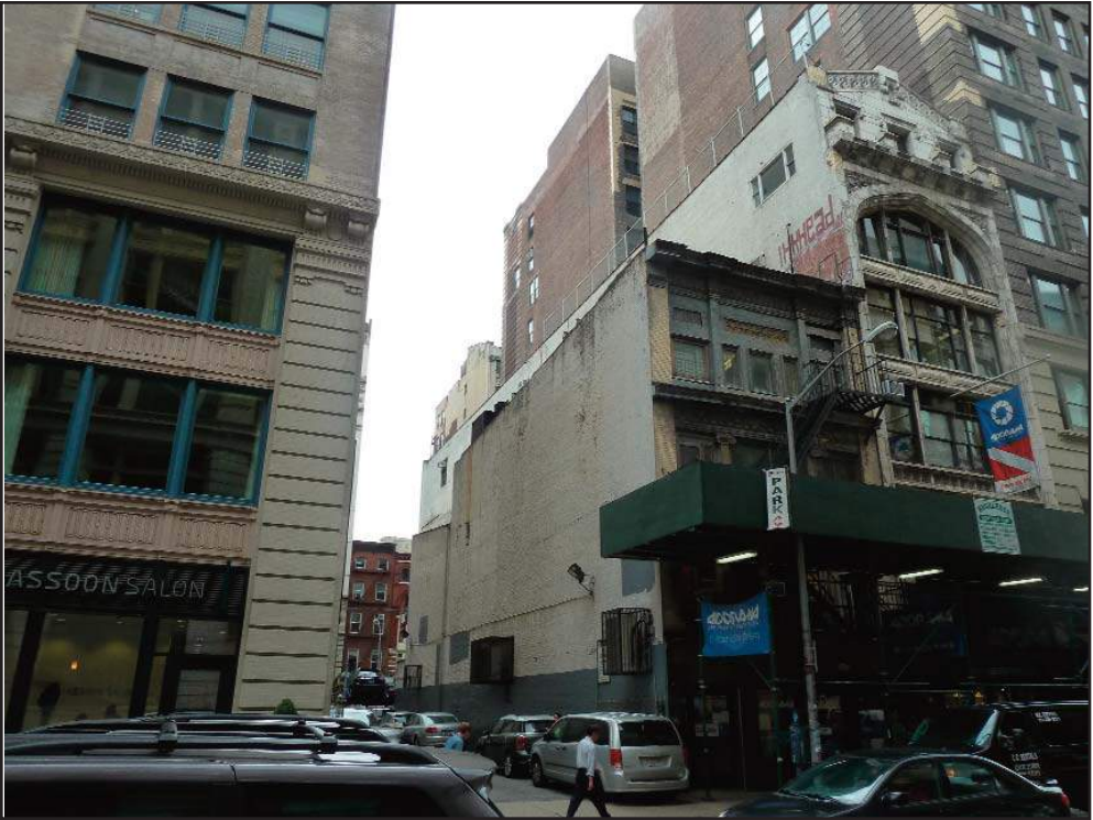
4. View from West 18th Street looking southwest - Lot 15 in center of photo (parking lot), existing buildings on Lot 66 and Lot 14 to the right.
