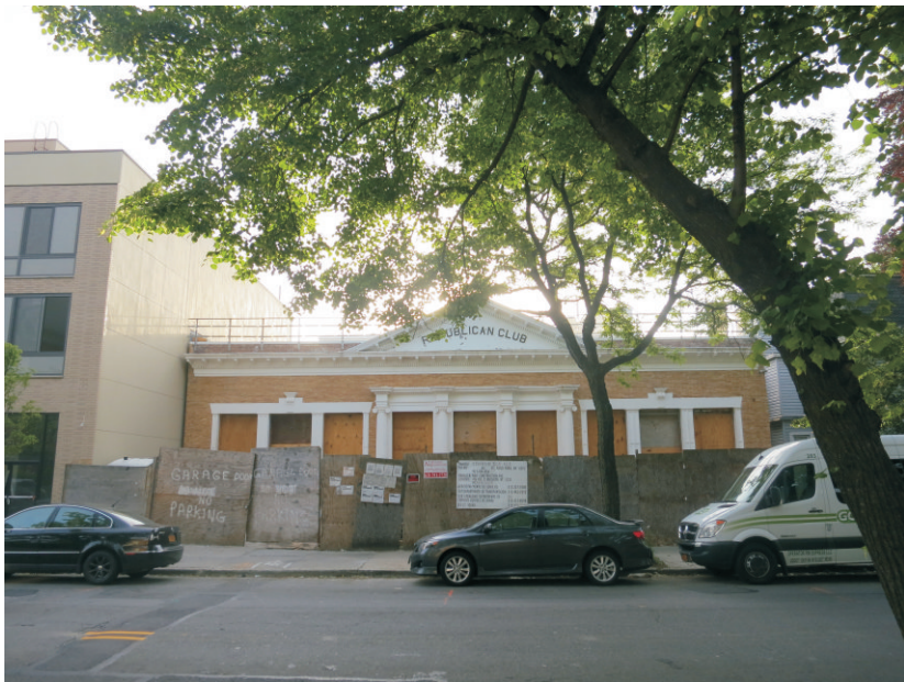
3. View of the Site, facing east.
