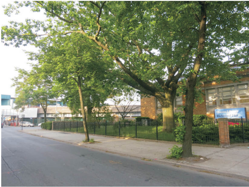
7. View of the Richmond Hill branch of the Queen Library (opposite the Site), facing southwest.
