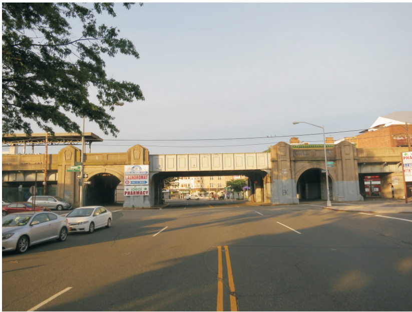
19. View of Hillside Avenue, facing southeast towards the LIRR overpass.
