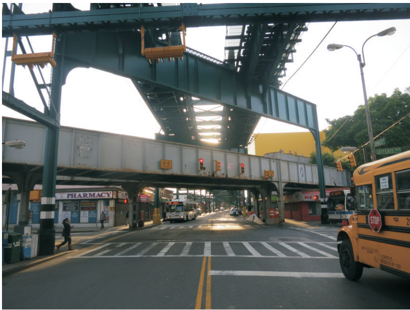
37. View of Jamaica Avenue, facing east from Lefferts Boulevard.
