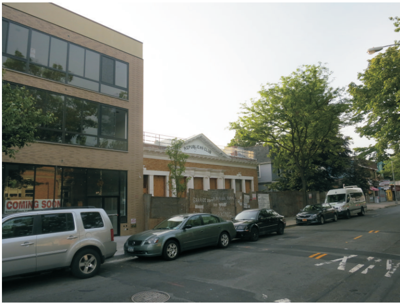
4. View of the Site, facing southeast.
