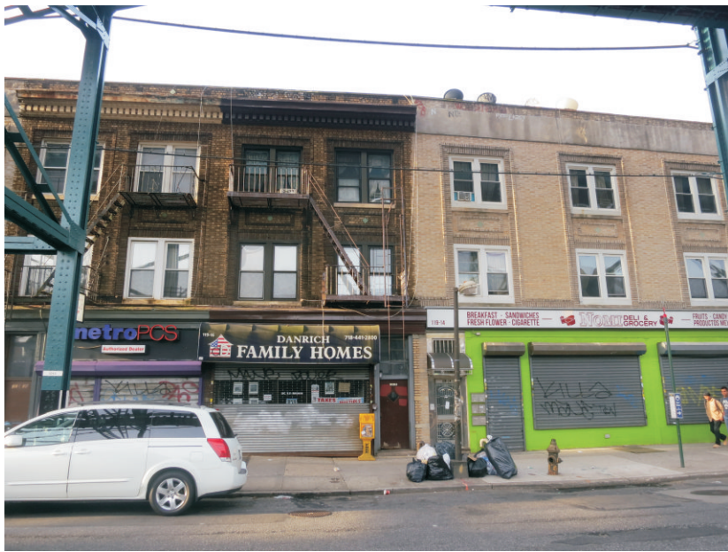
13. Mixed use building on the south side of Jamaica Avenue just east of Lefferts Boulevard.
