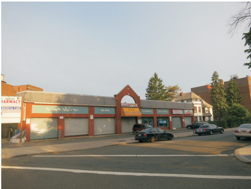
21. View of the retail strip on the west corner of Hillside Avenue and 118th Street.
