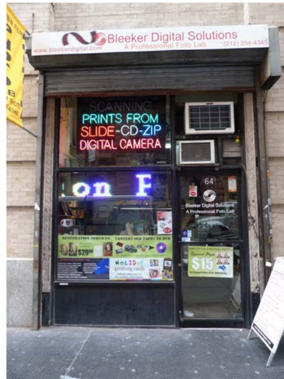
Non-historic Storefront Infill at Photo Store on Blecker Street
