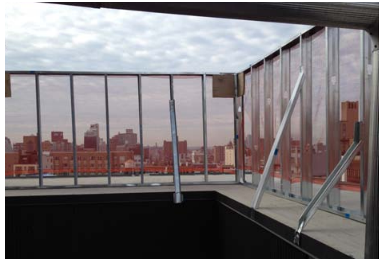
Mock-up of Balustrade installed on North and West Roof Parapet
