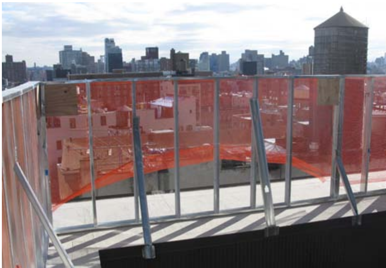
Mock-up of Balustrade installed on North and East Roof Parapet
