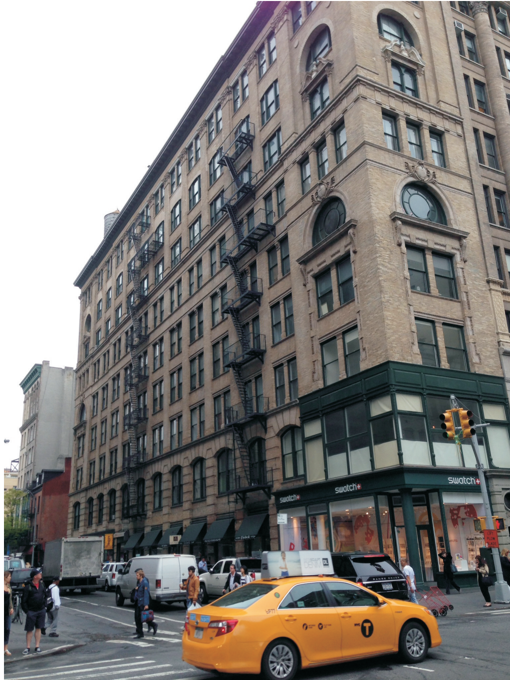
Frontage of building along Bleeker Street between Broadway and Crosby Street
