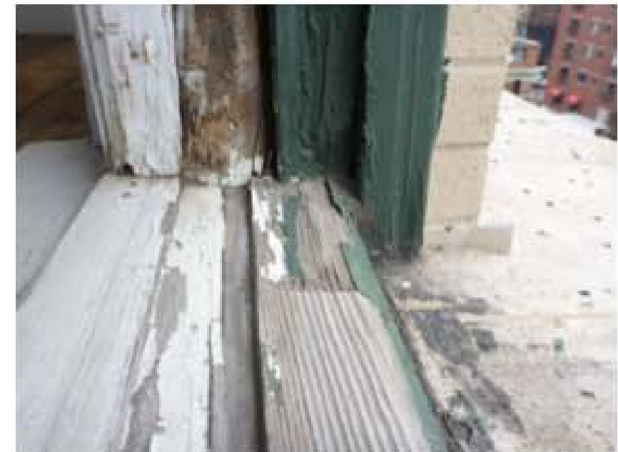
TYPICAL WINDOW - EXISTING CONIDITIONS
