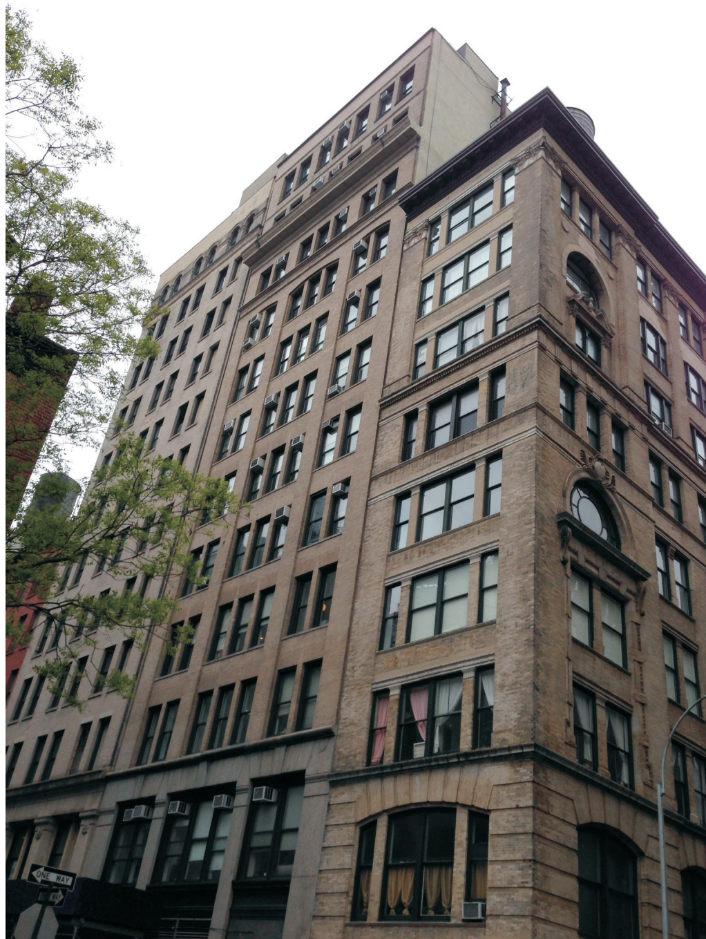
Frontage of building at the southwest corner of Bleecker and Crosby Streets
