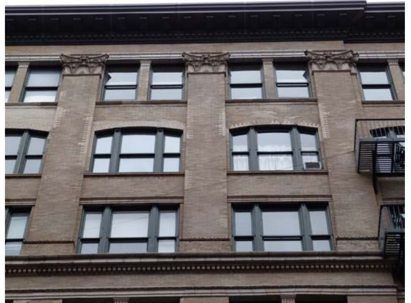
Masonry Repairs and New Copper Cornice on Bleecker Street
