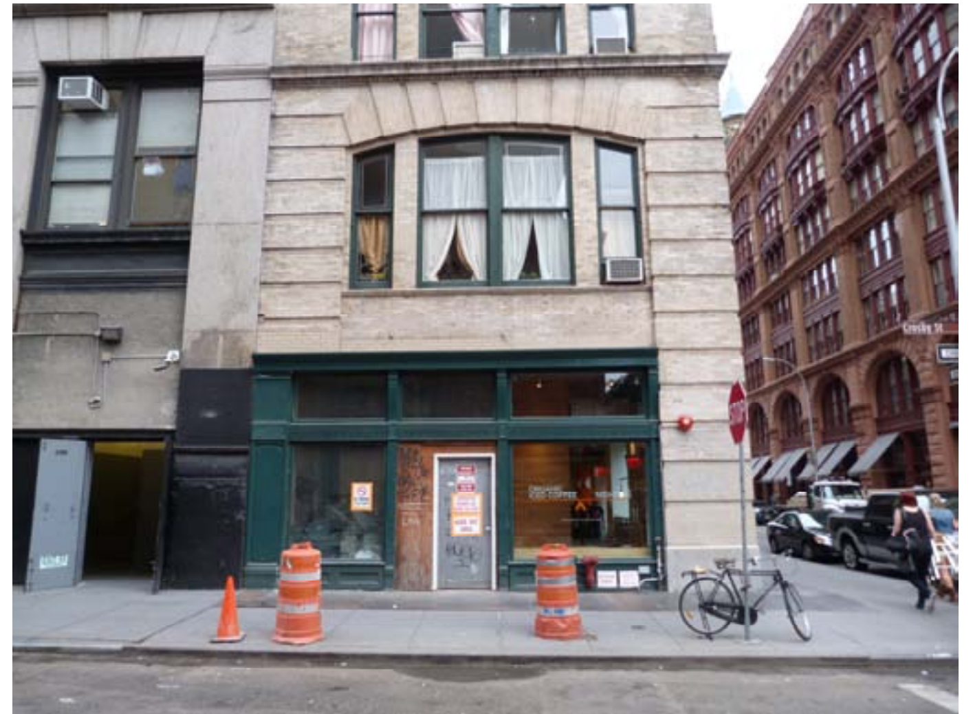
Storefront Repairs in Progress on Crosby St.
