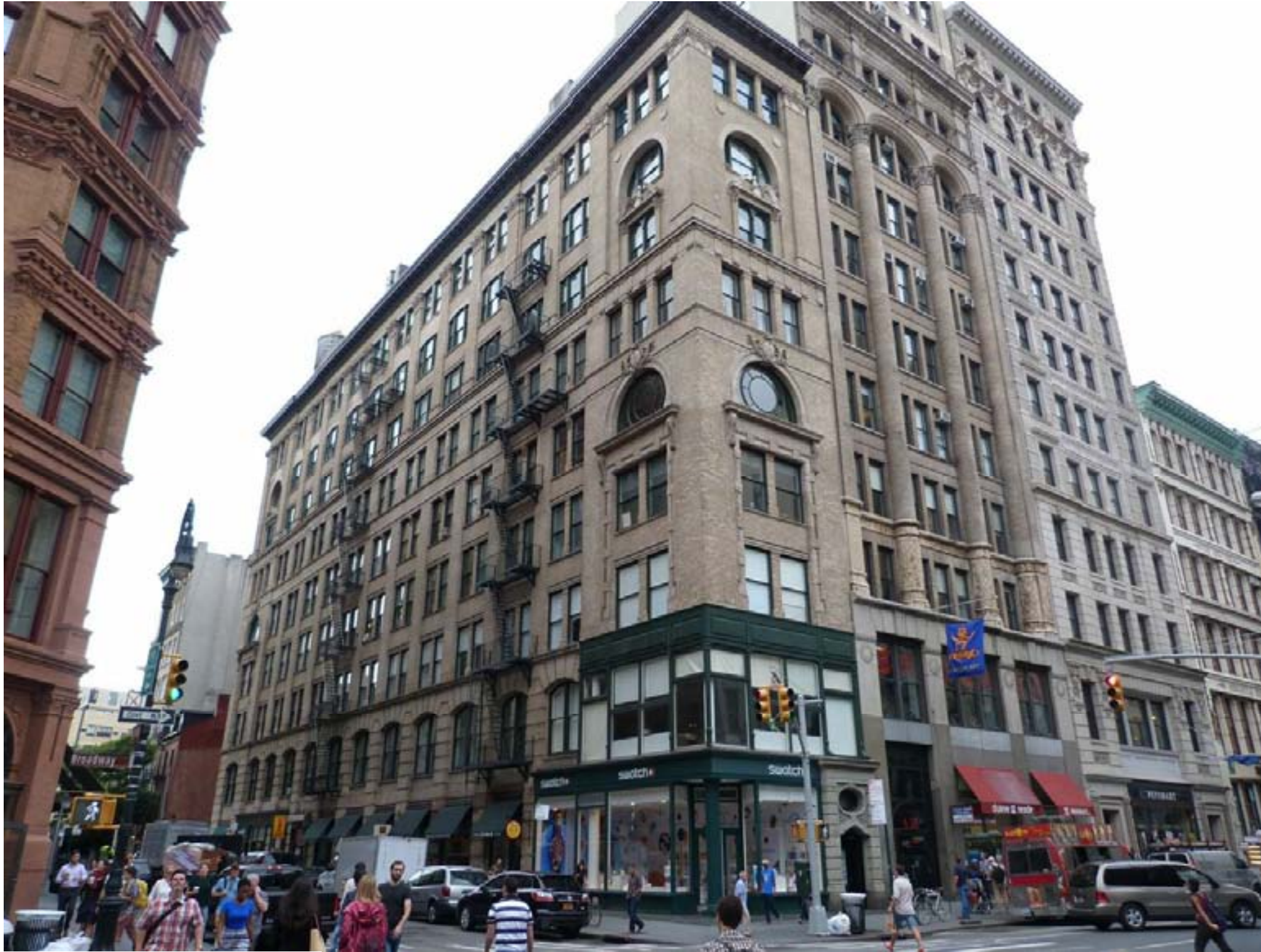
Present Condition, View Southeast
