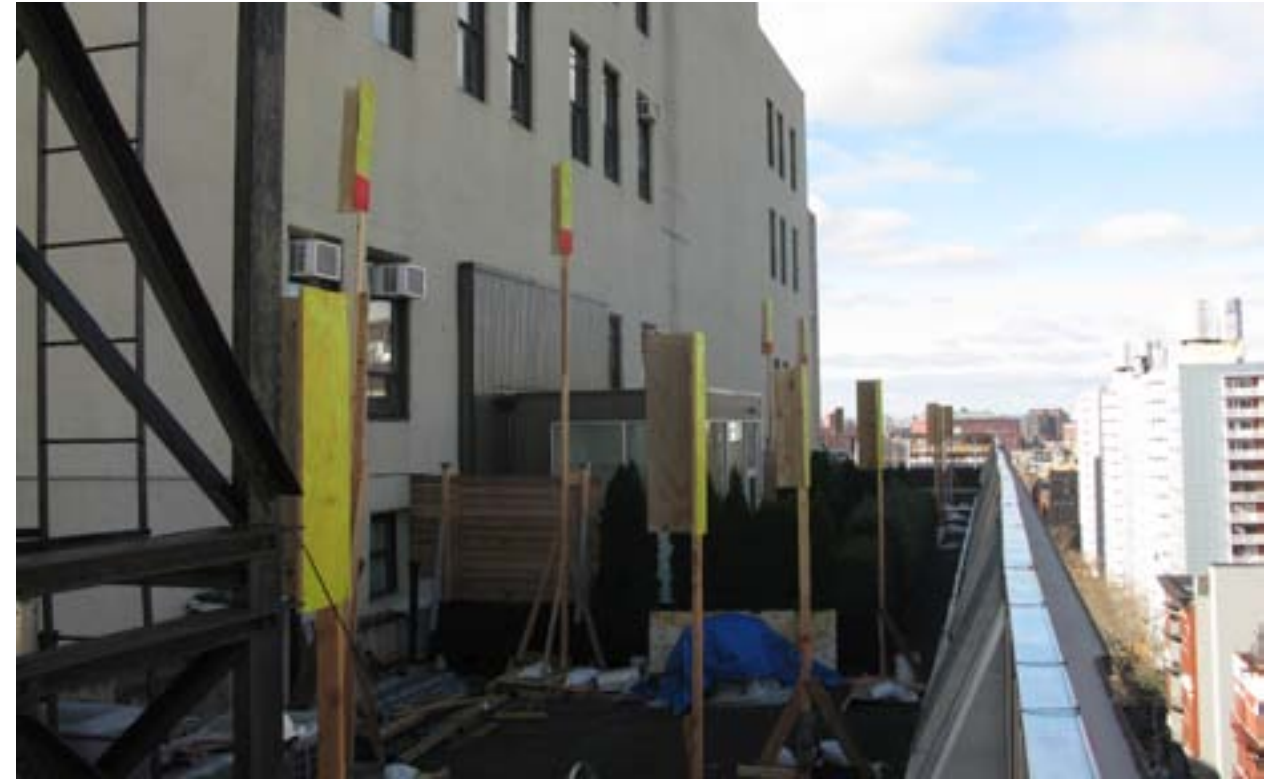
Mock-up Marker Posts installed on West Side of Main Roof
