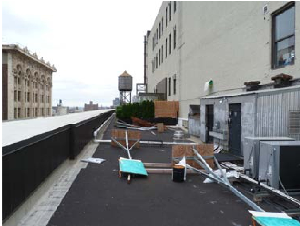
View of Roof Looking East
