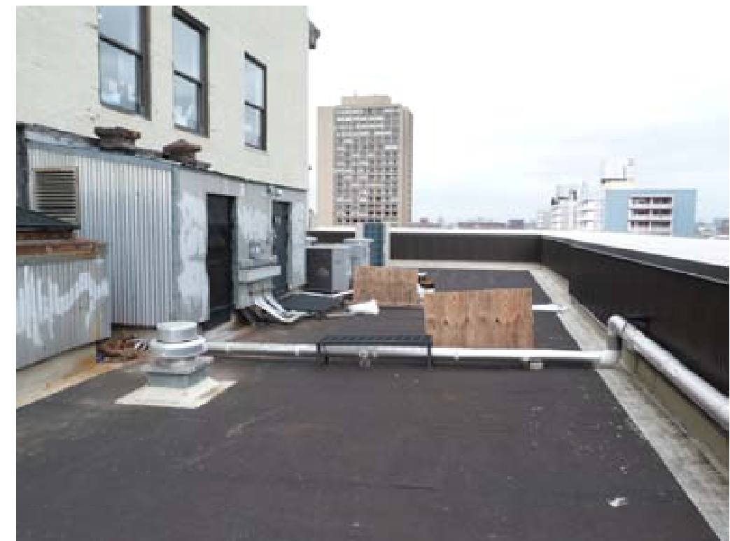
Bulkheads, and Pipes on west end of roof
