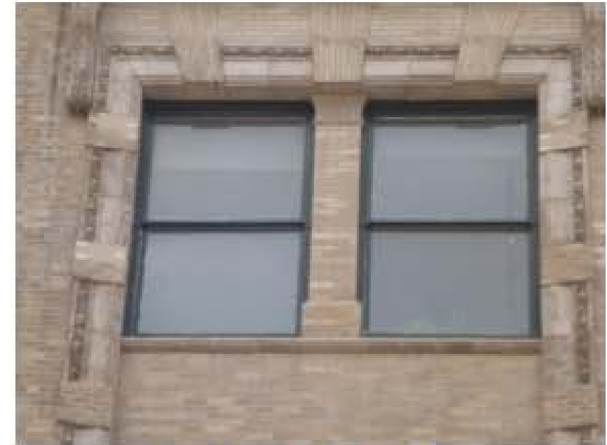
TYPICAL WINDOW - EXISTING CONIDITIONS
