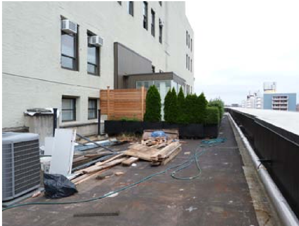
View of Roof Looking West
