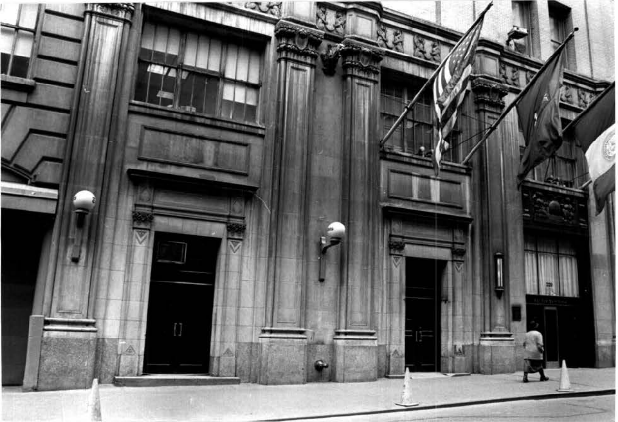
New York Times Building (originally Times Annex) 43 rd Street facade, first story, center Photo: Carl Forster
