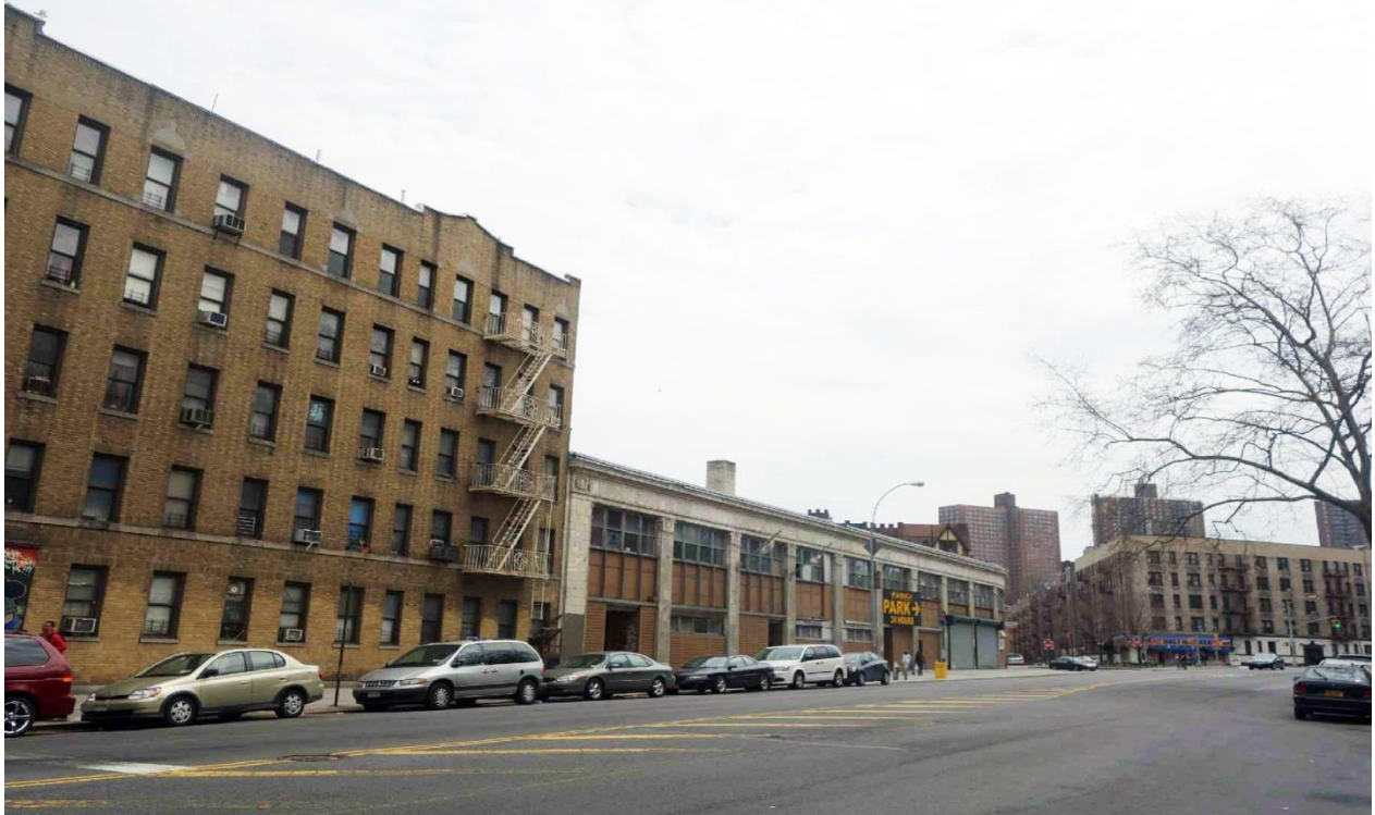
Photograph 5: Entrance to Fort Tryon Park (looking southeast at Project Site - 2014)
