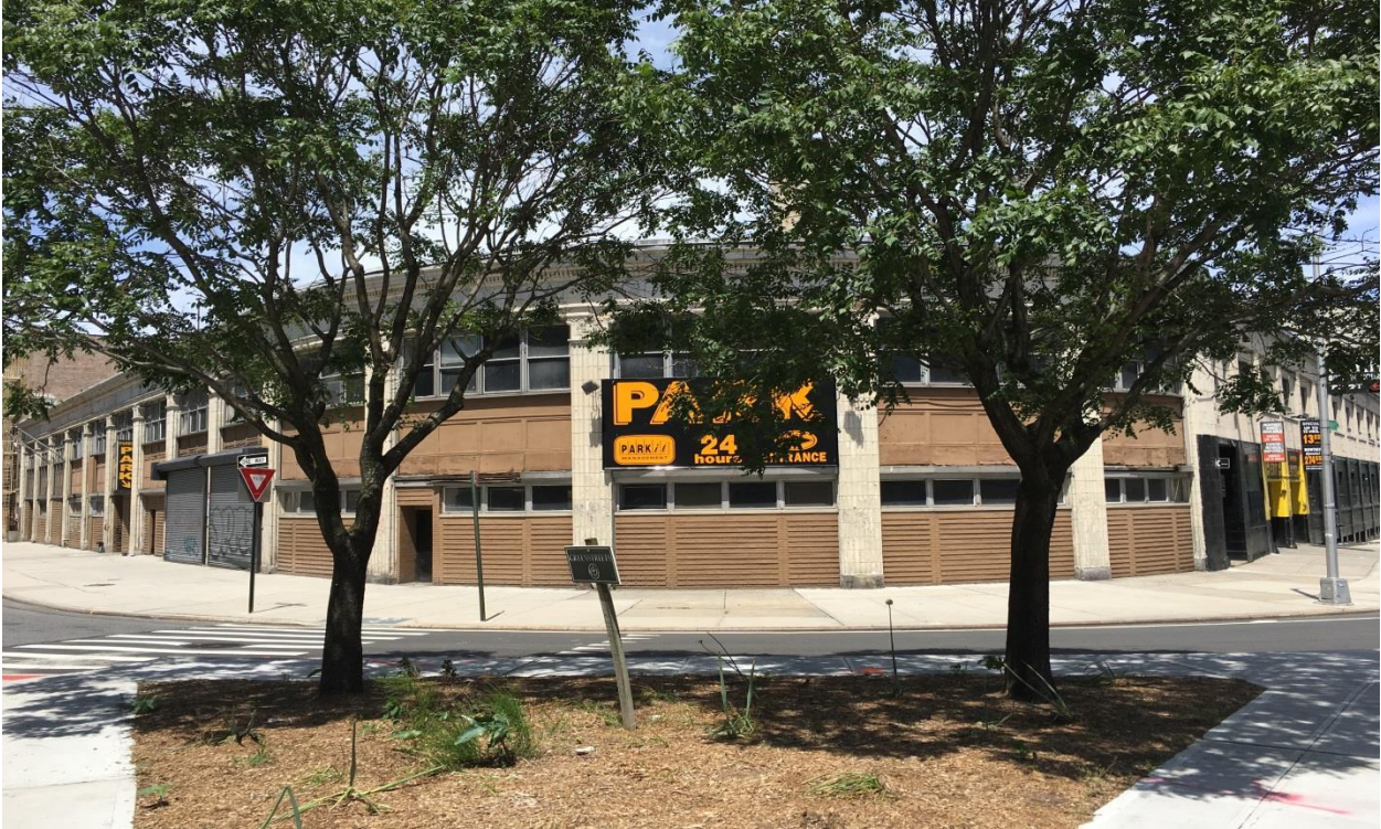
Photograph 1: Broadway and Sherman Avenue (looking northeast at Project Site -2016)
