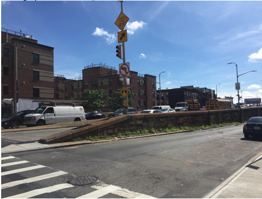
View of Atlantic Avenue Bridge adjacent to Projected Site 1 looking northeast
