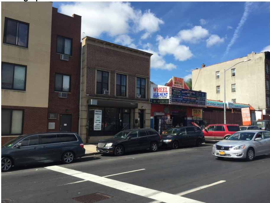
View of Projected Site 2 and adjacent lots on Atlantic Avenue
