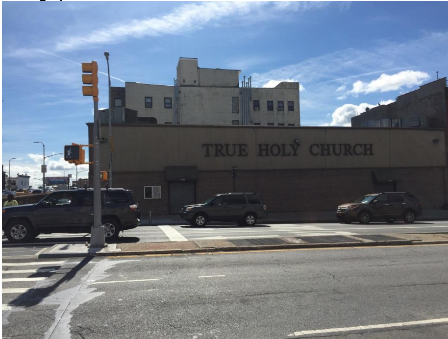
View of Projected Site 1 at 1860 Eastern Parkway
