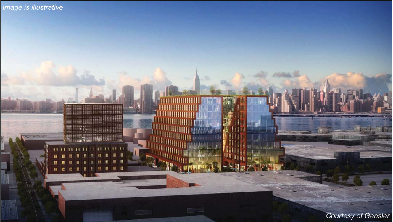
6. With-Action Condition: View northwest of proposed project.
