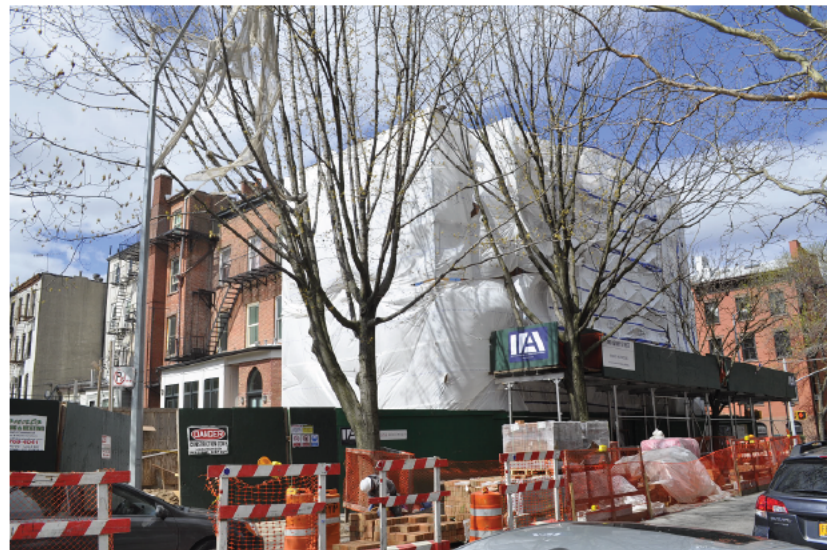
A - LOOKING SOUTHWEST ALONG KANE ST
