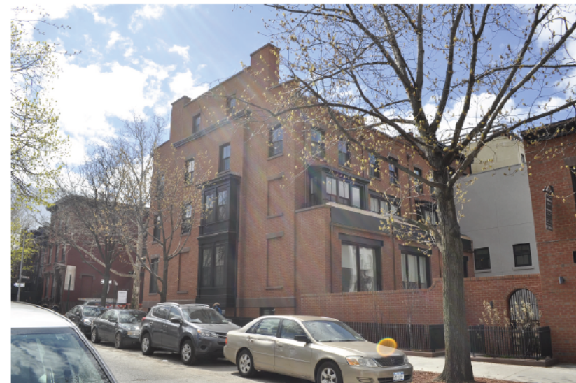
E - LOOKING SOUTHEAST ALONG KANE ST
