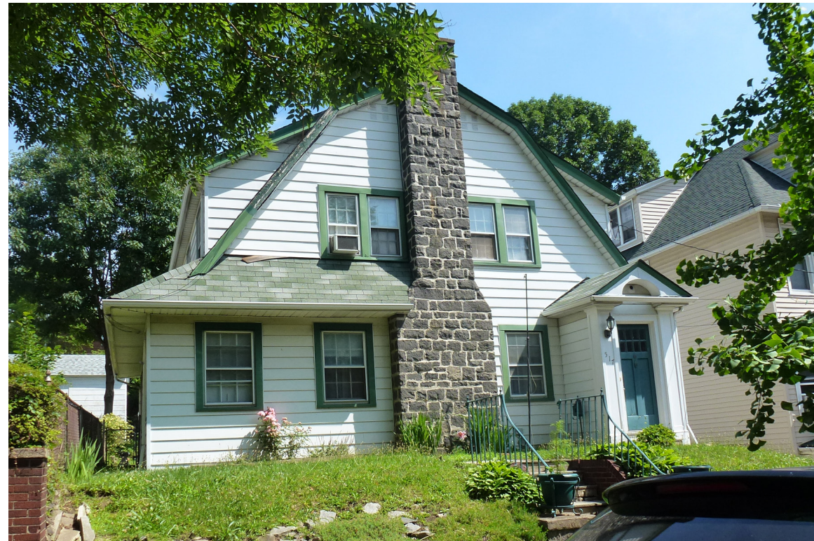
1. Looking north from E. 236th Street Photo taken: 6.19.15
