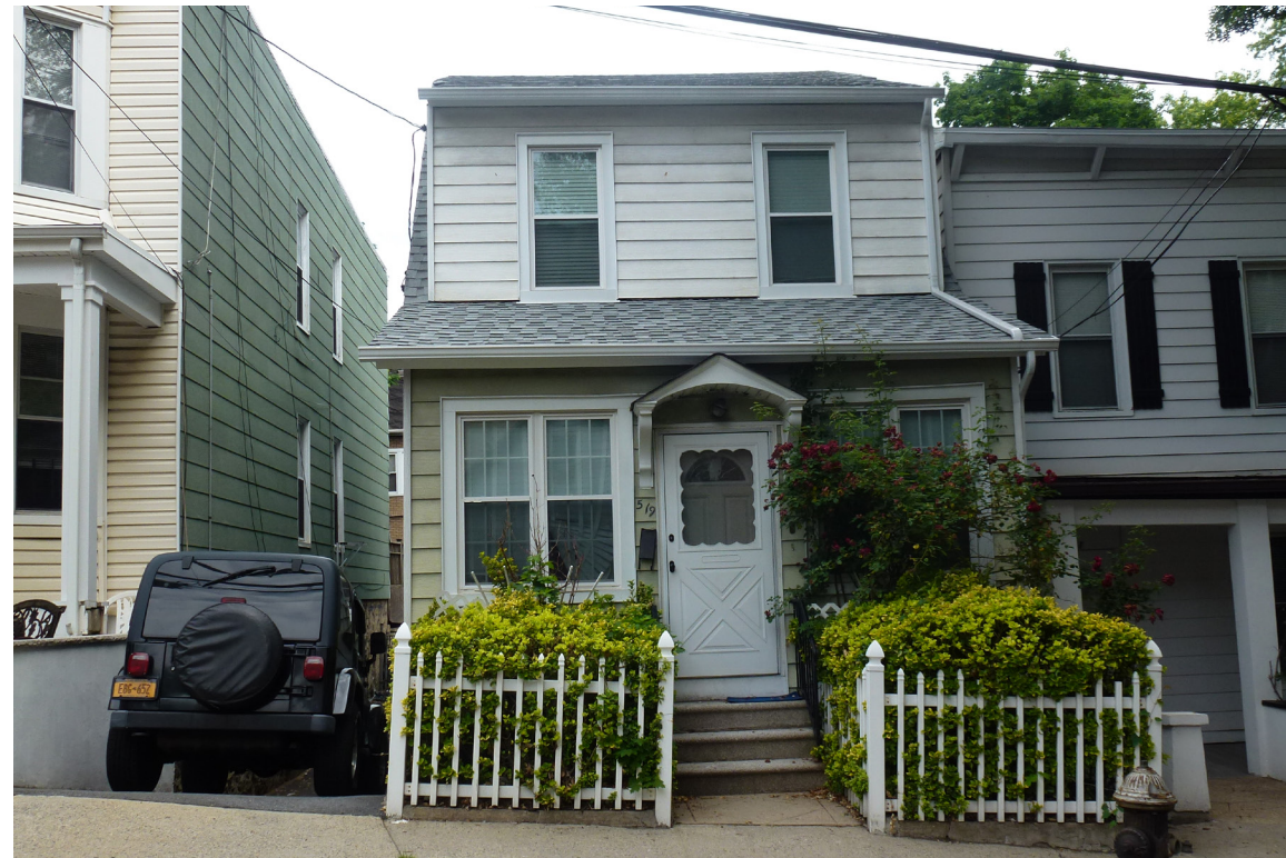
1. Looking north from E. 235th Street Photo taken: 6.19.15
