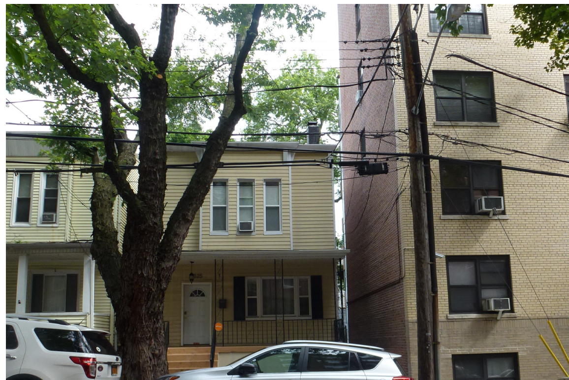
3. Looking north from E. 235th Street Photo taken: 6.19.15
