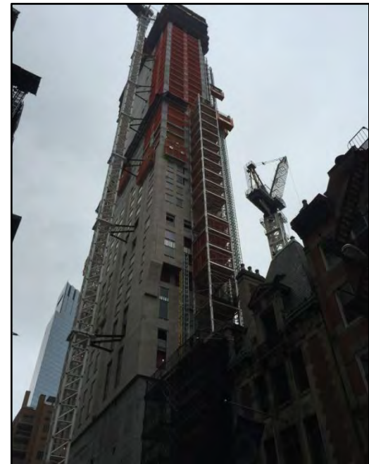
4. View northwest of the 220 CPS development from W.58th Street.
