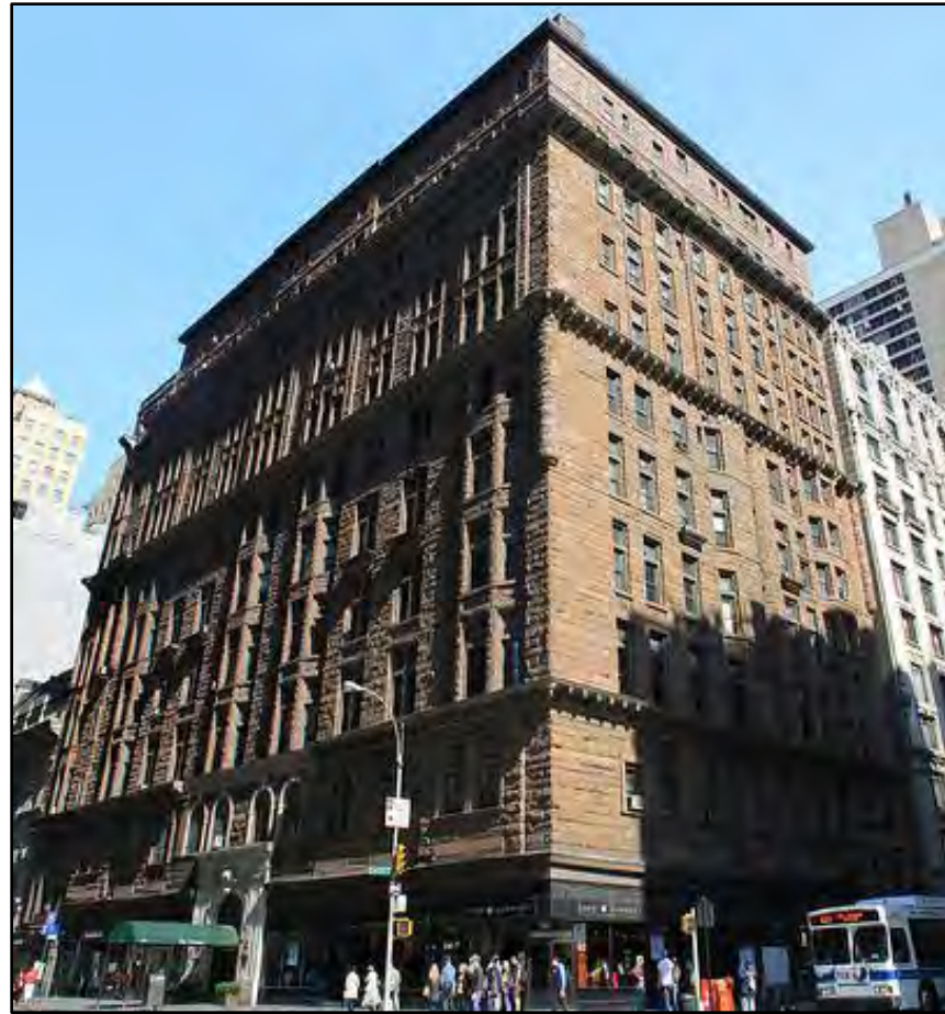
8. Osbourne Apartments (205 W. 57th Street).
