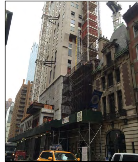
3. View northwest of the project site from W.58th Street.
