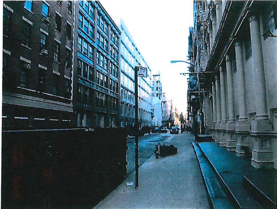
9. View Wooster Street from Canal Street
