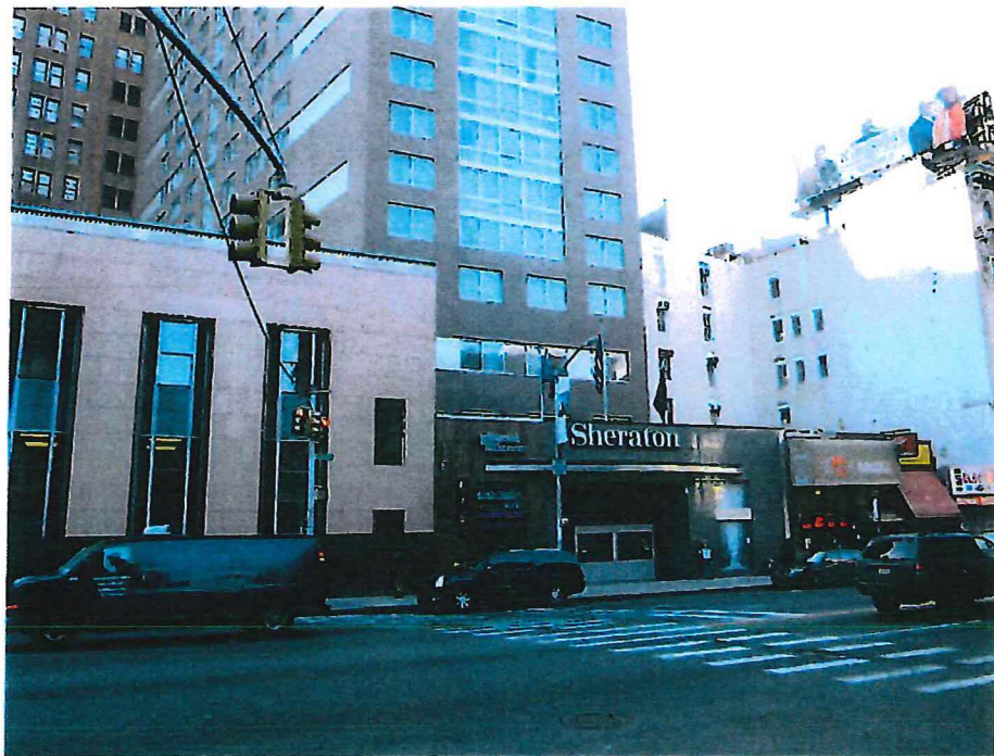
10. View South across Canal Street from corner of Wooster Street
