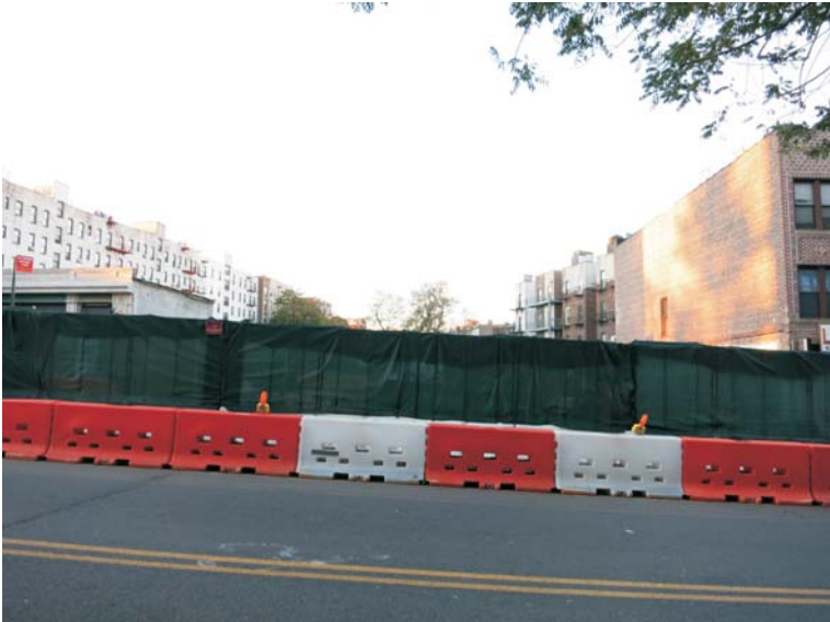
3. View of the Site facing north from Lincoln Road.
