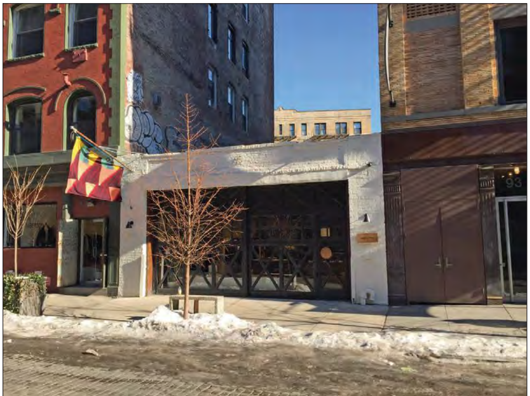
View of Adjacent Non-Contributing Building 2
