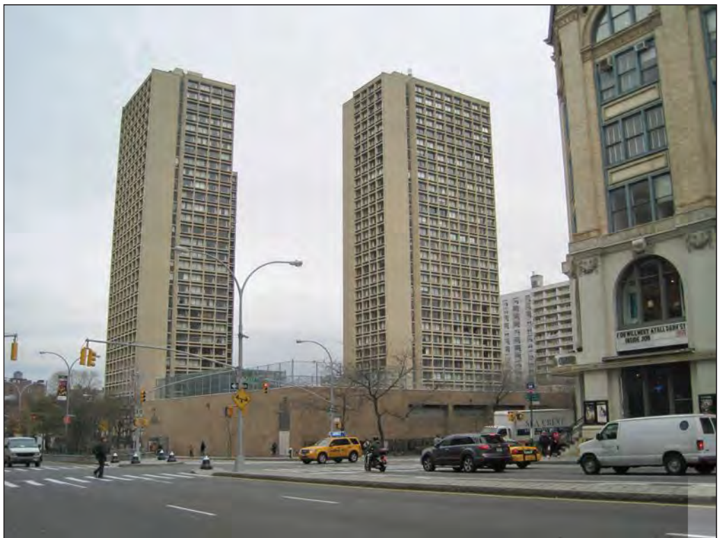
View of University Village from West Houston Street and Mercer Street 3
