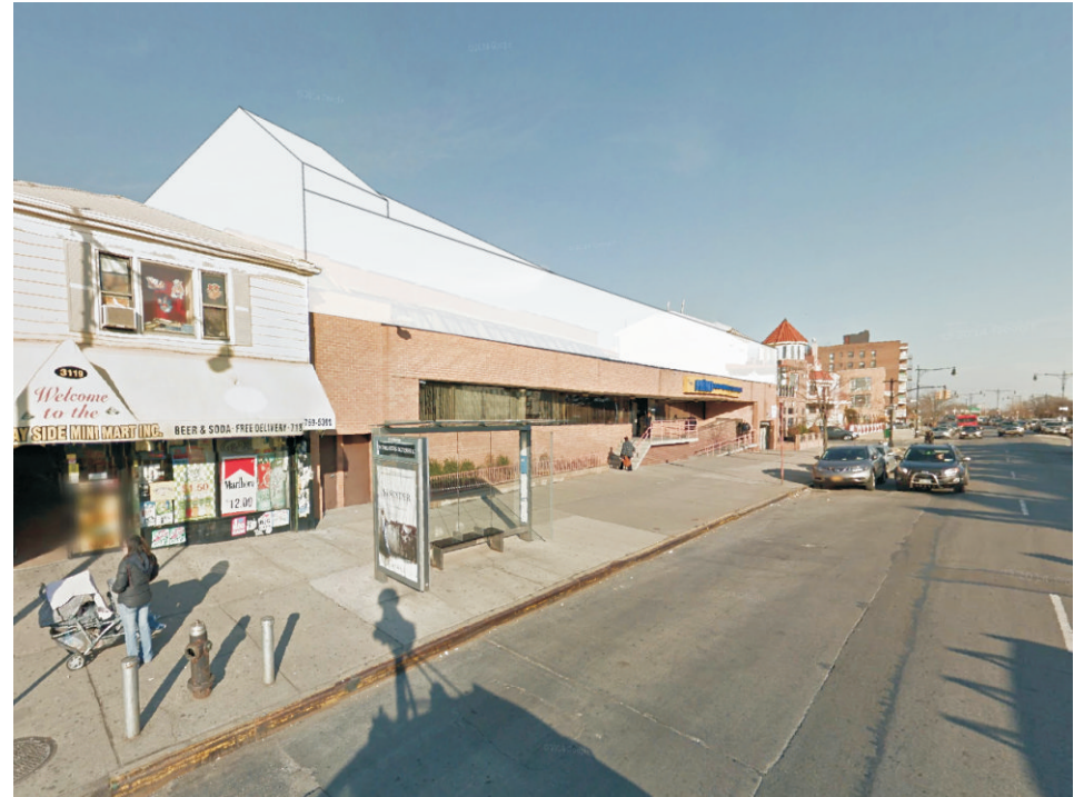
Emmons Avenue facing east toward the Site
