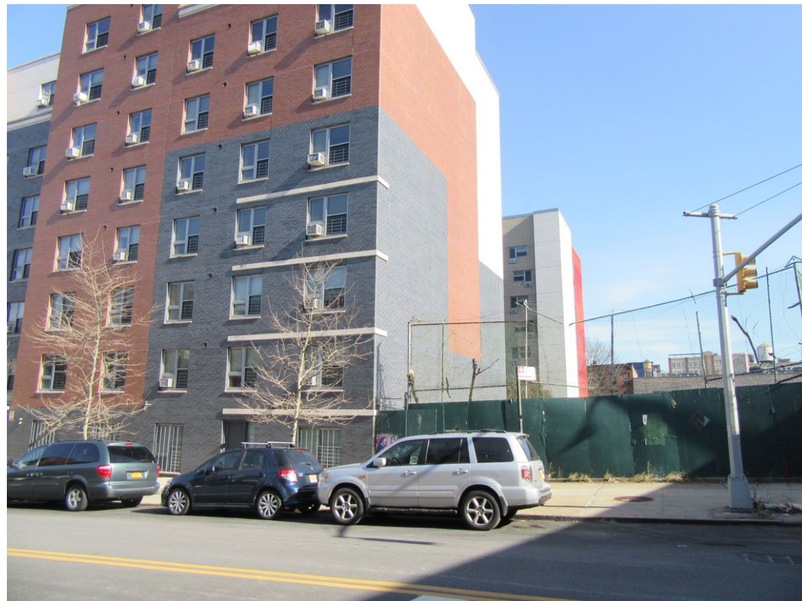
18. View of the east side of Clermont Avenue, facing northeast (Site at right).
