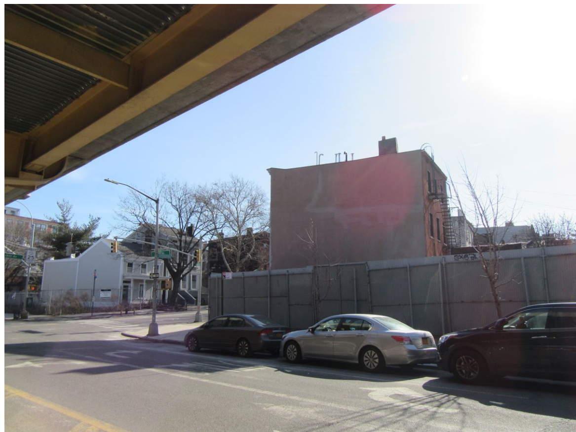
9. View of the south side of Park Avenue, facing southeast.
