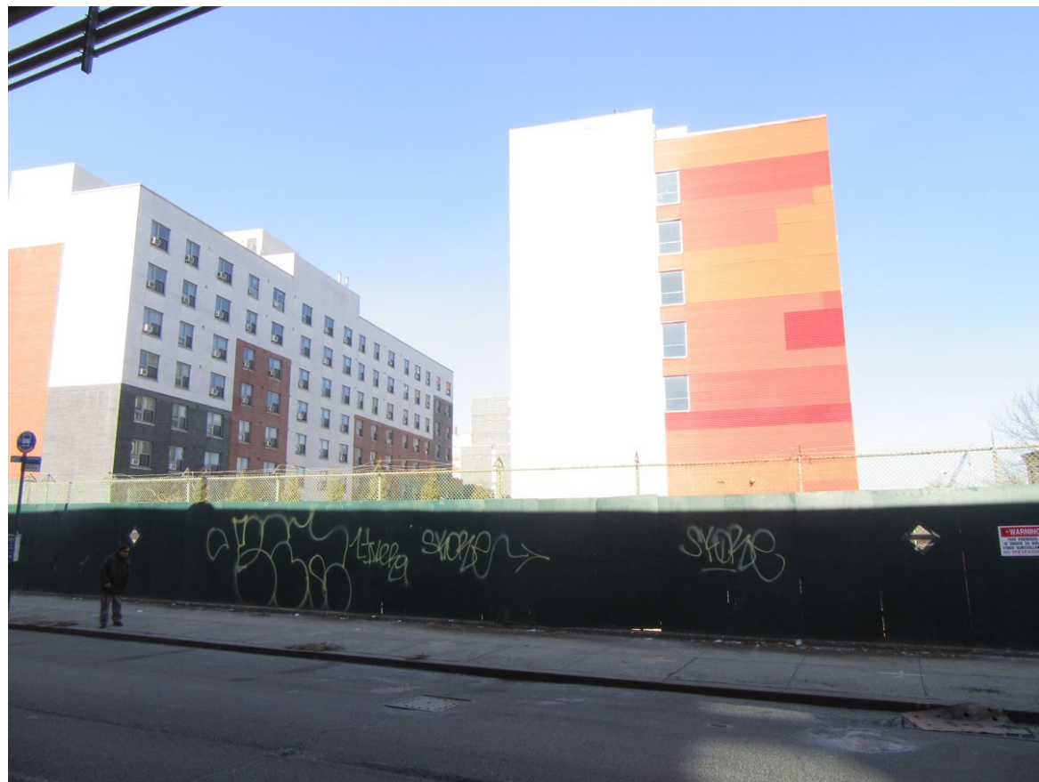
7. View of the Site from Park Avenue, facing northwest.
