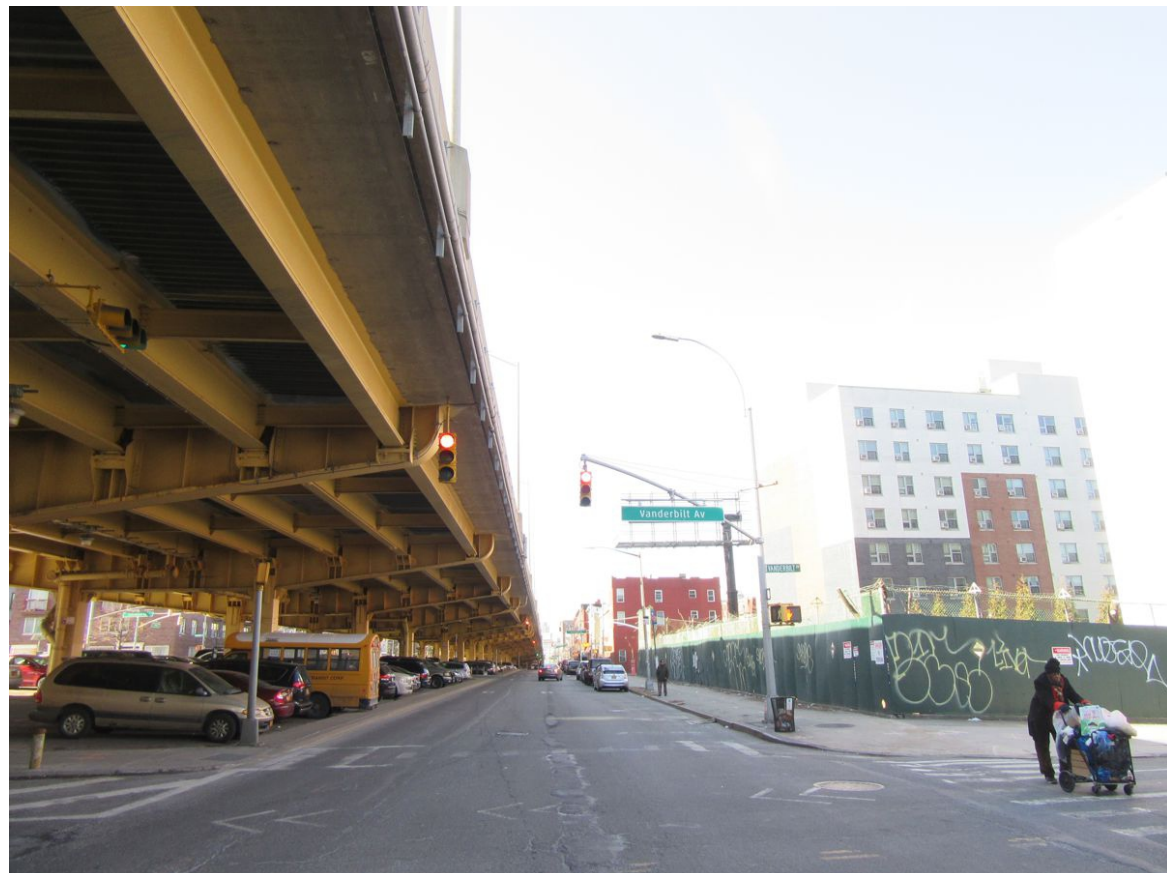
6. View of the north side of Park Avenue, facing west (Site at right).
