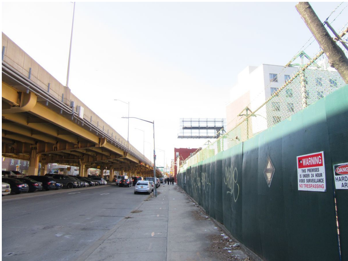
21. View of the sidewalk along the north side of Park Avenue facing west from Vanderbilt Avenue (Site at right)
