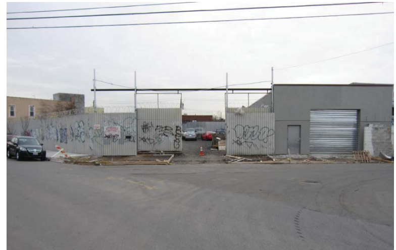
11 - VIEW OF PROPERTY BEHIND DEVELOPMENT SITE FROM INTERSECTION OF HART PLACE AND WEST 16TH STREET
