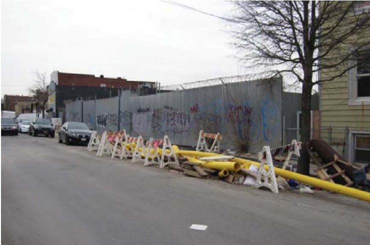
01 - VIEW OF DEVELOPMENT SITE LOOKING SOUTHWEST FROM ACROSS WEST 15TH STREET
