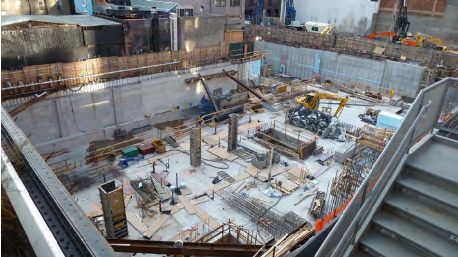
6. View of Development Site looking southwest from High Line access stairs
