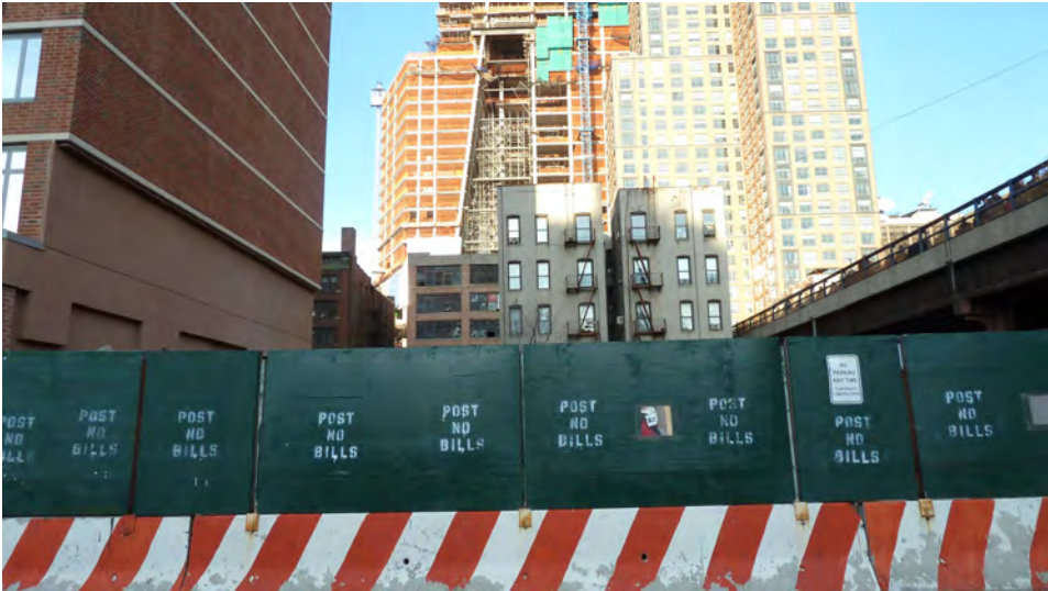
7. View looking north on W 28th Street
