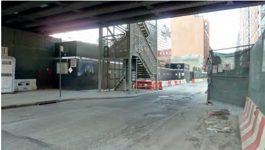
1. View of Development Site looking southwest from W 28th Street with High Line overhead
