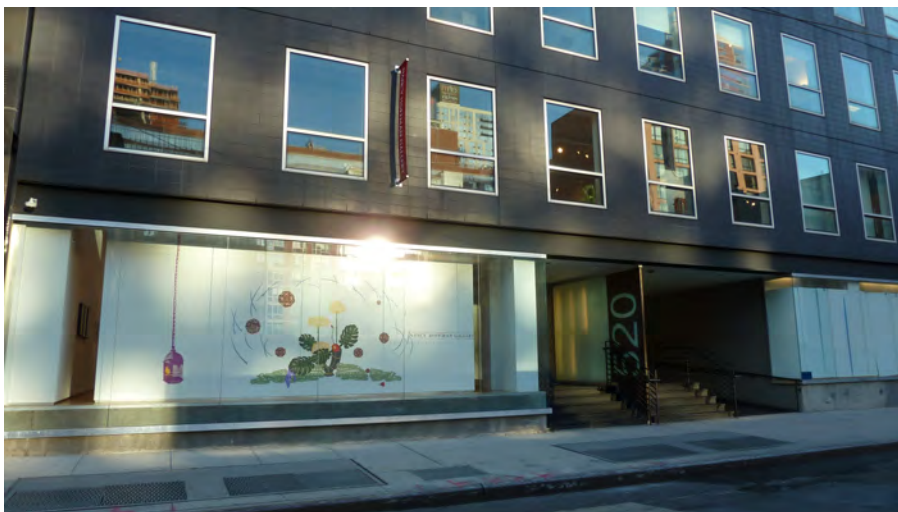
11. View from Development Site looking south from W 27th Street
