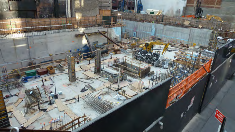
5. View of Development Site looking southwest from High Line access stairs
