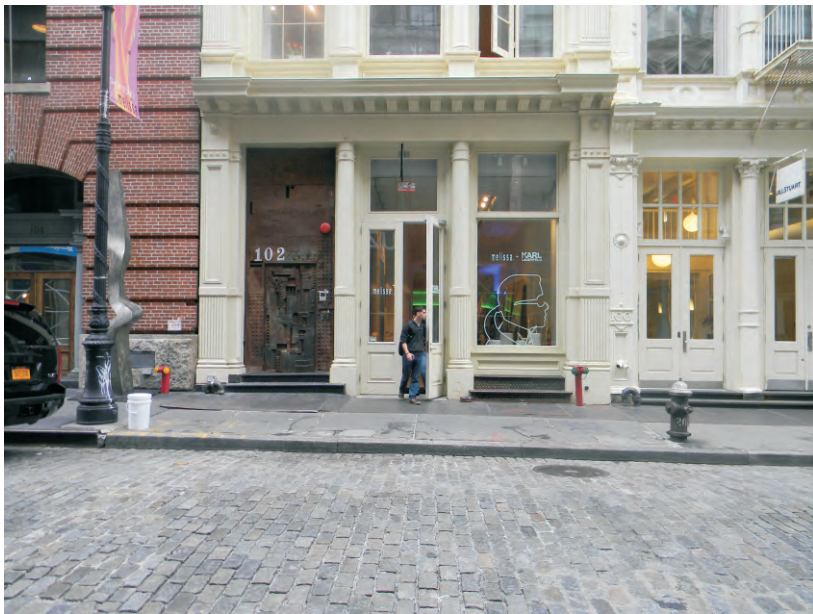
15. 102 Greene Street (the Site) (Block 499, Lot 6)
