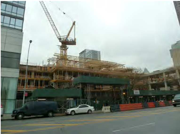
3. Southwest corner of site
