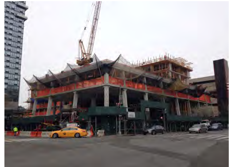
4. Southeast corner of site
