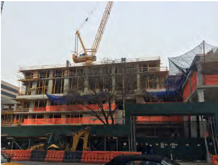
7. View of site looking north
