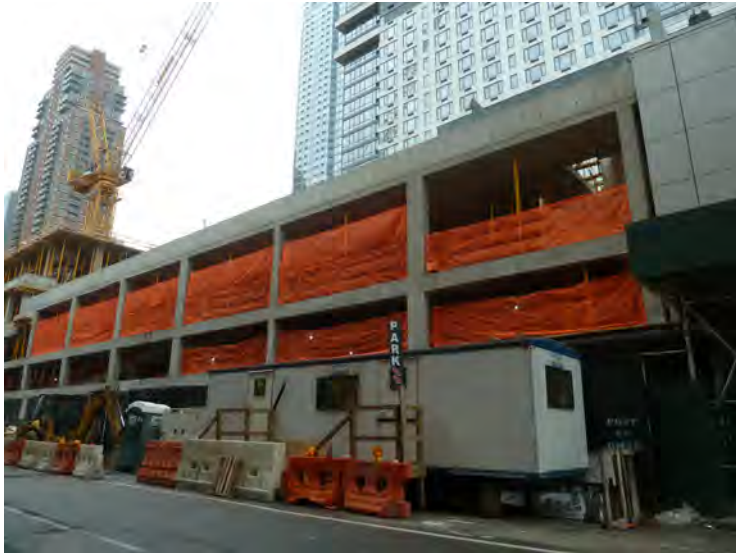
5. View of site looking south
