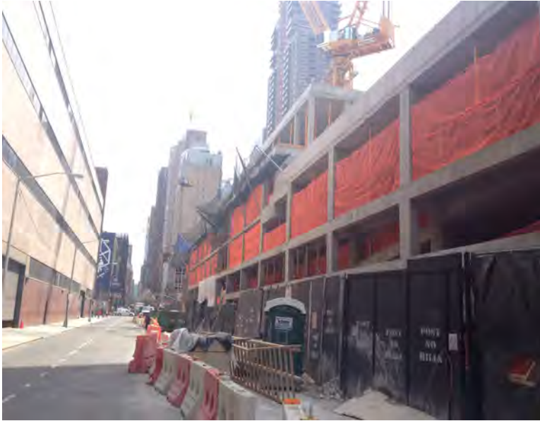
1. Northwest corner of site
