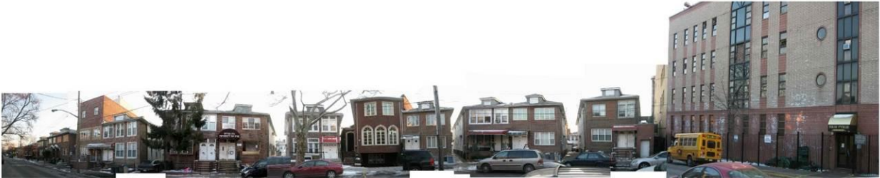
Photo D-4: 54 th Street Elevation East of FortHamilton Parkway, Looking South
