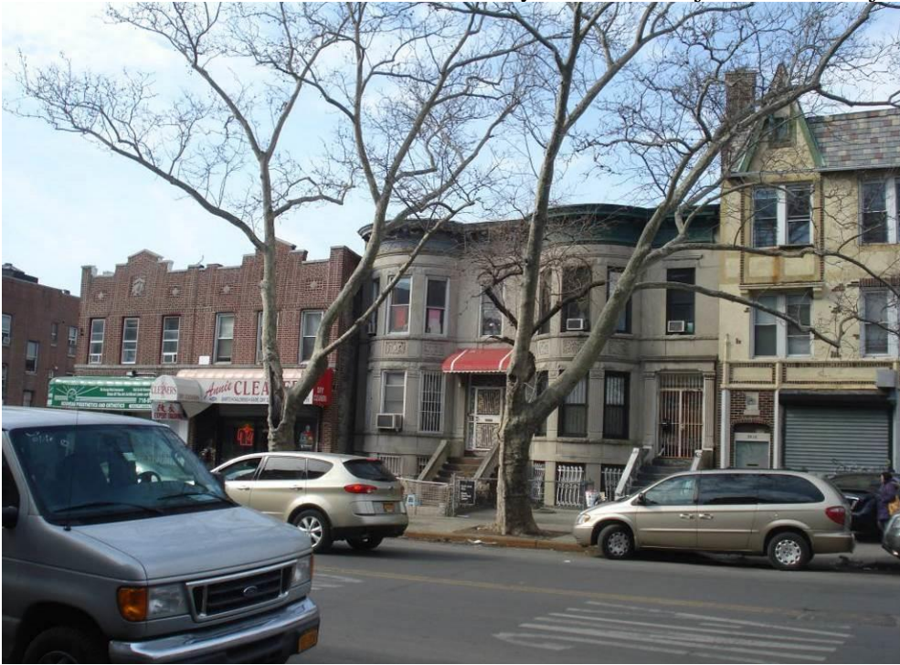
Photo D-6: View West to Fort Hamilton Parkway Blockfront Adjacent to the Project Site
