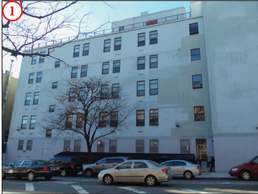
View of the northeast corner of the project site.
