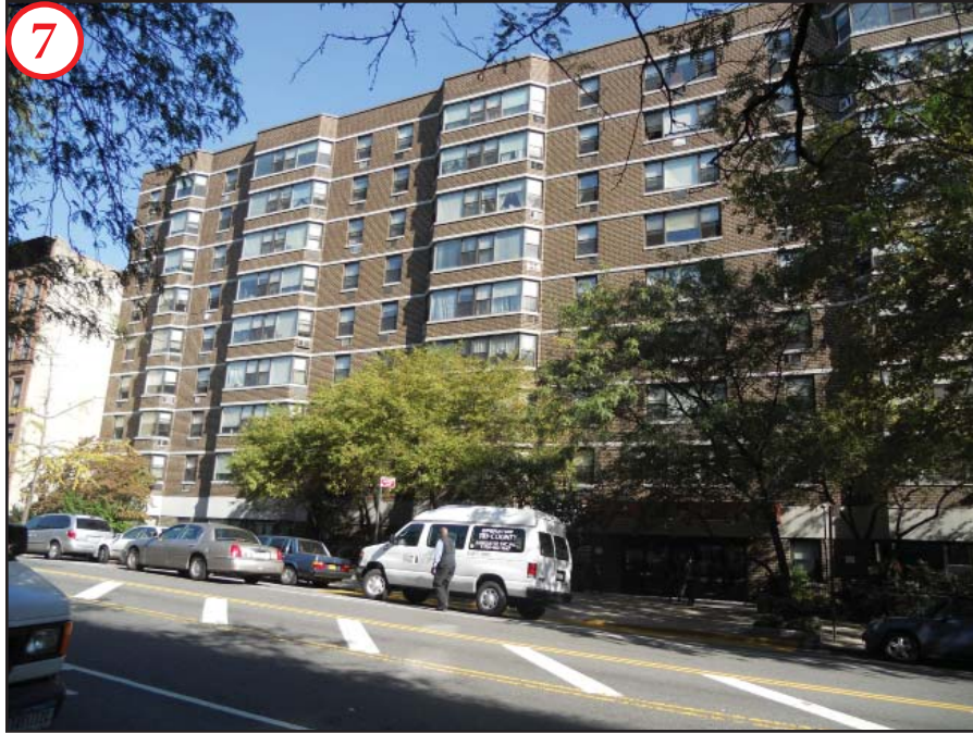
View north across West 106th Street from the project site.
