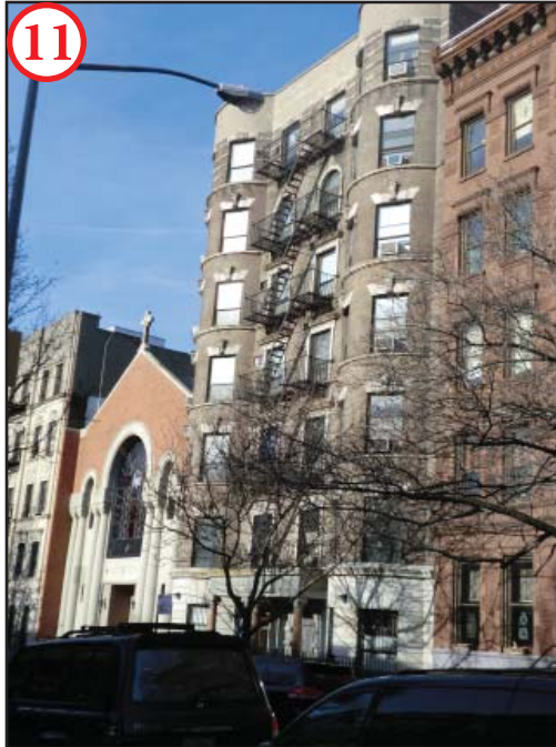
View northwest of the north side of West 105th Street.
