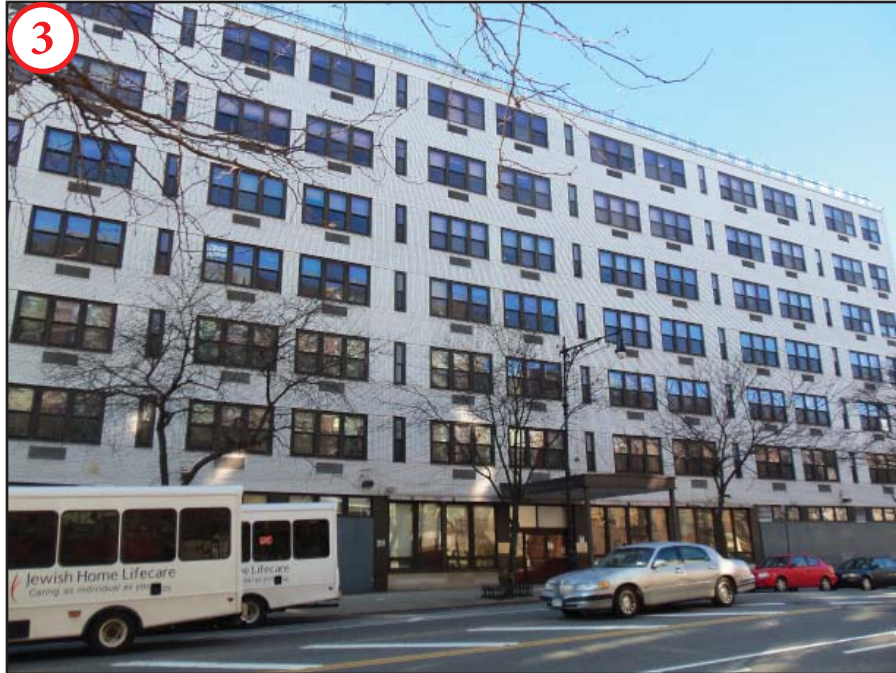
View of project site frontage along 106th Street.
