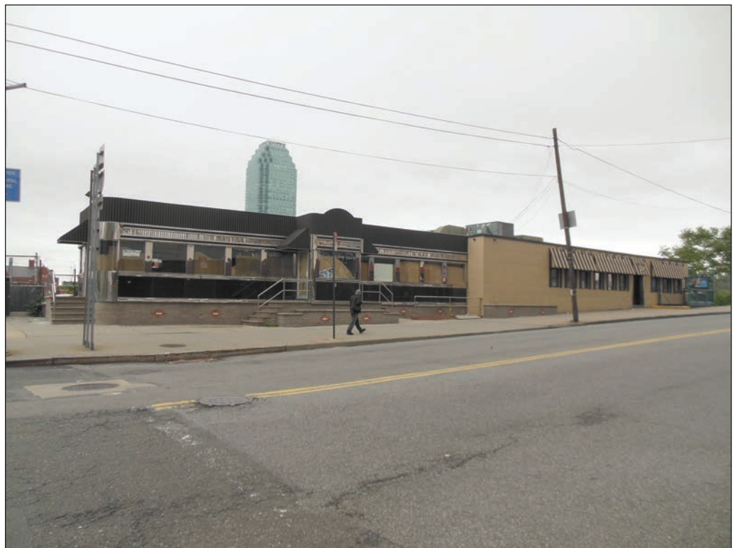
View of former Blue Sky Diner and addition 4
