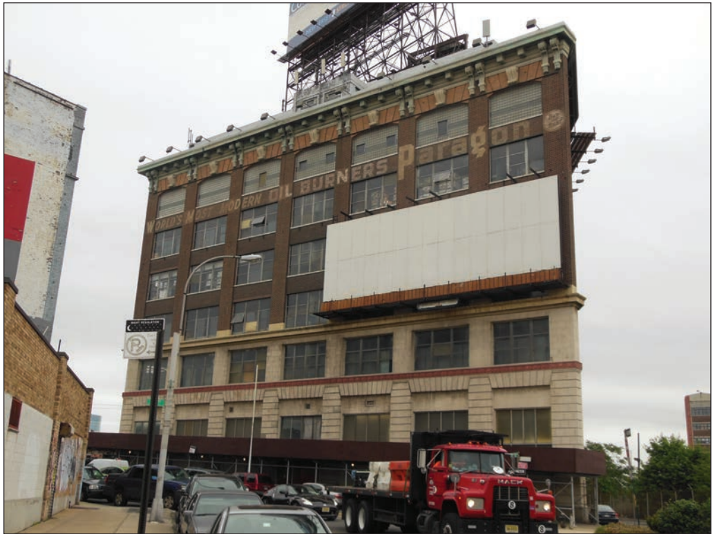
View of west façade of Paragon Oil building 2
