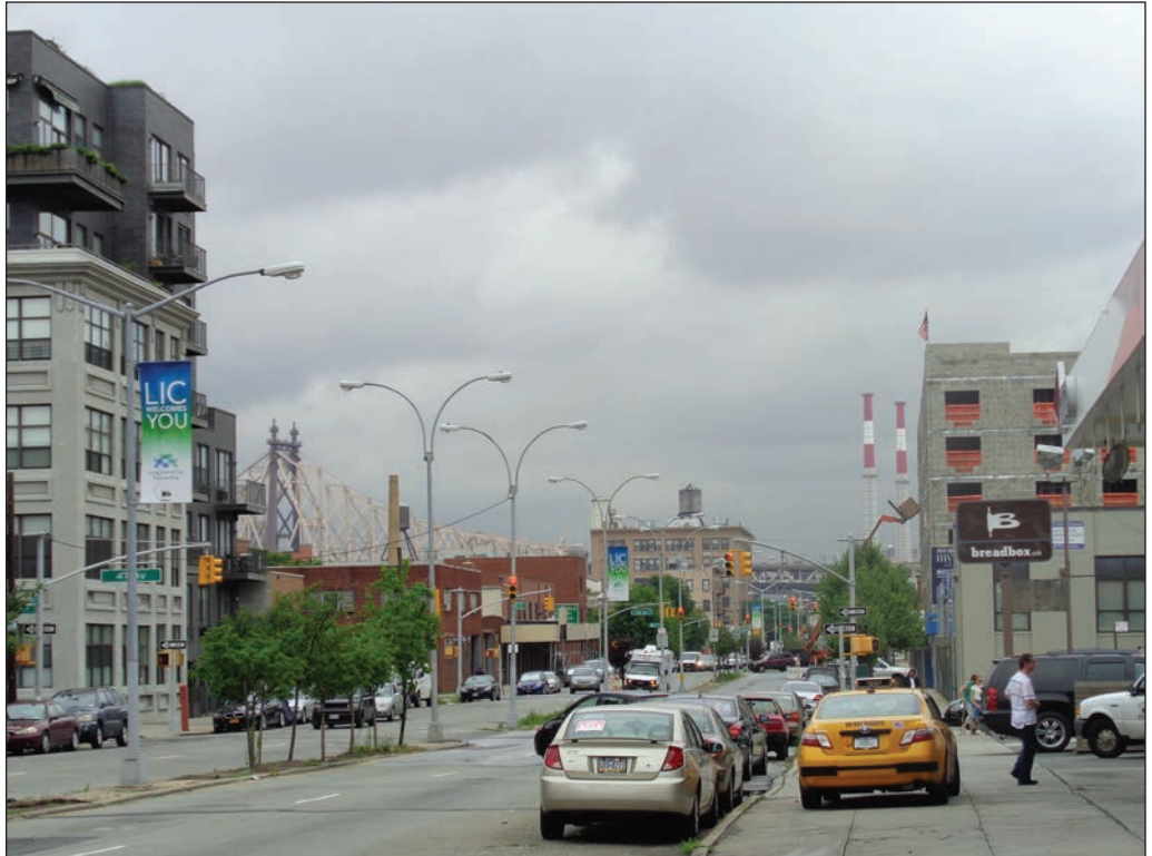
View northwest of the tower, span, and trusswork of the Queensboro (59th Street) Bridge and the smokestacks of the "Big Allis" Power Plant 23
