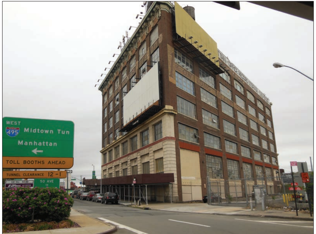
View of south façade of Paragon Oil building 3
