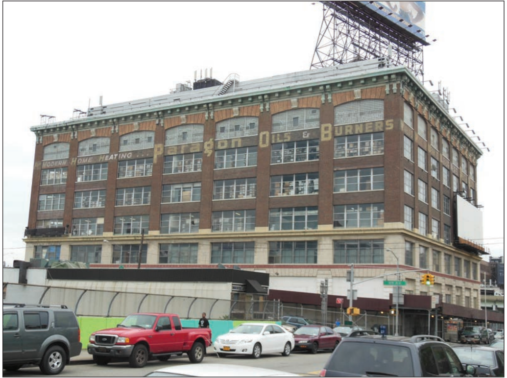
View of north façade of Paragon Oil building 1
