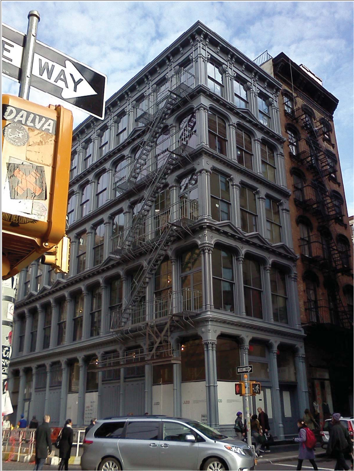
5. Northeast Corner Spring Street at Mercer Street
