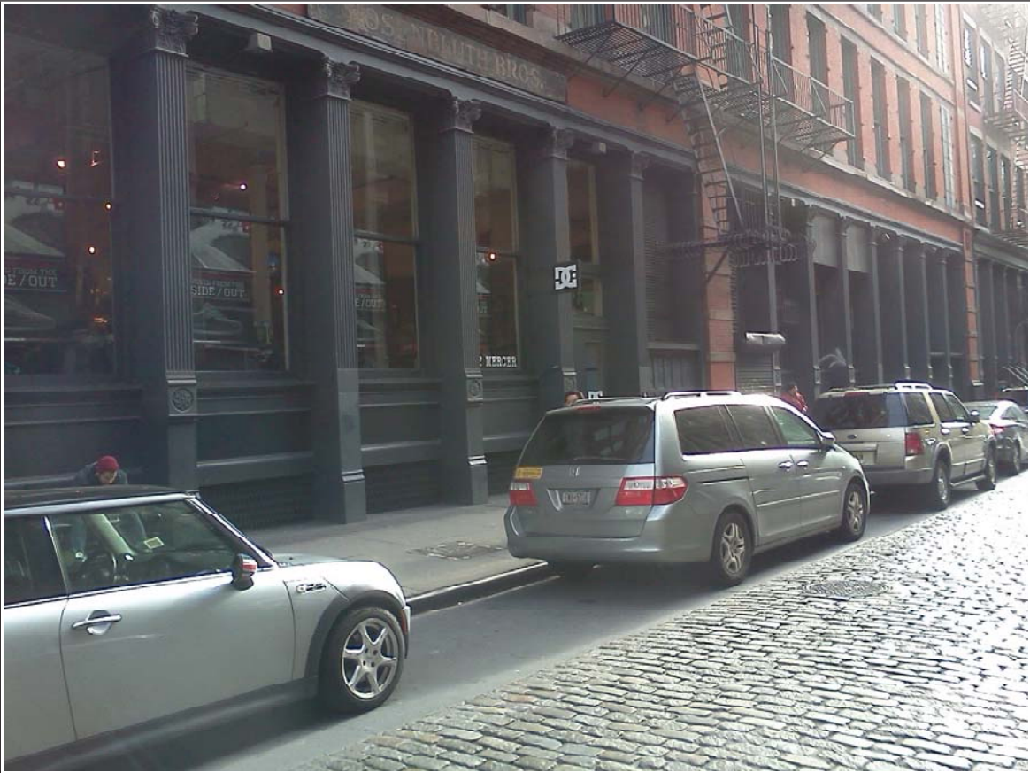
7. East Side of Mercer Street Facing South
