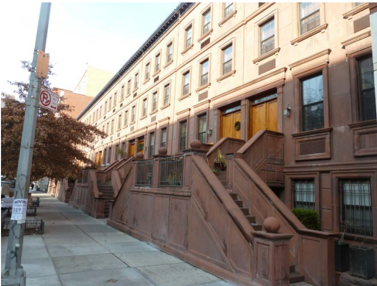
West 117 th Street west of Frederick Douglass Boulevard
