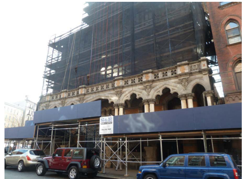
8. Vacant church building (Lot 14) on West 118 th St.
