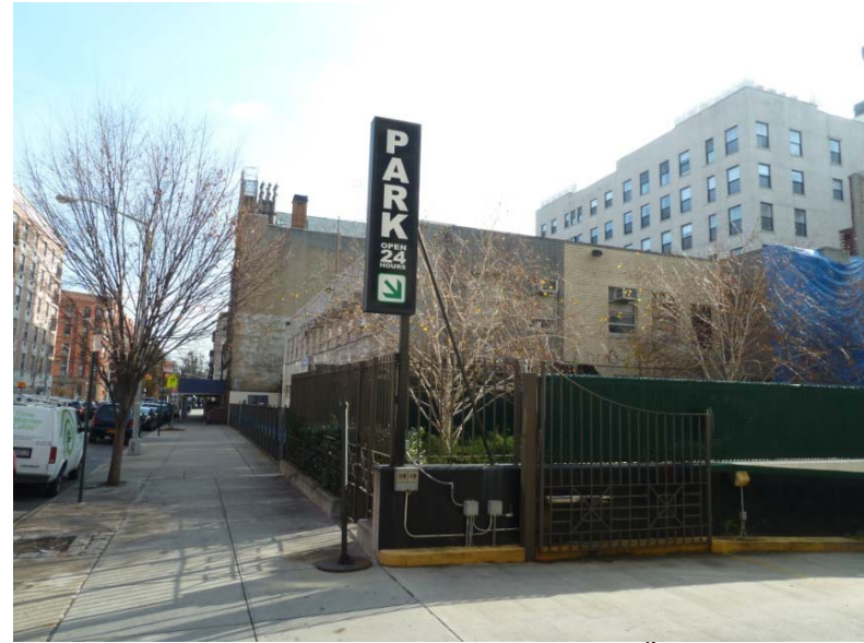
Sidewalk conditions along West 118 th Street
