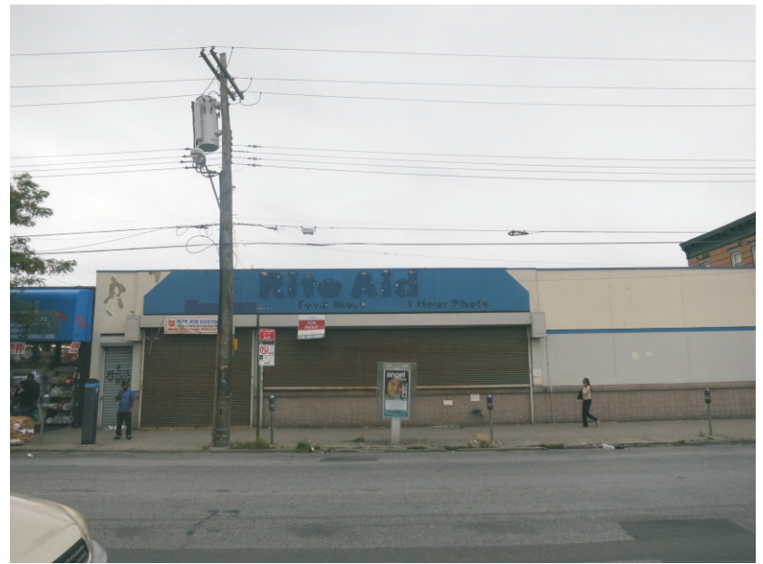
2. View of the Site, facing southwest.
