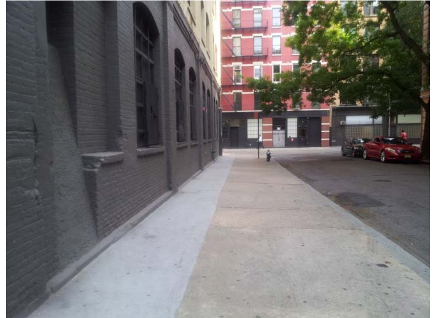
2 Looking north along the Mott St. frontage of the building
