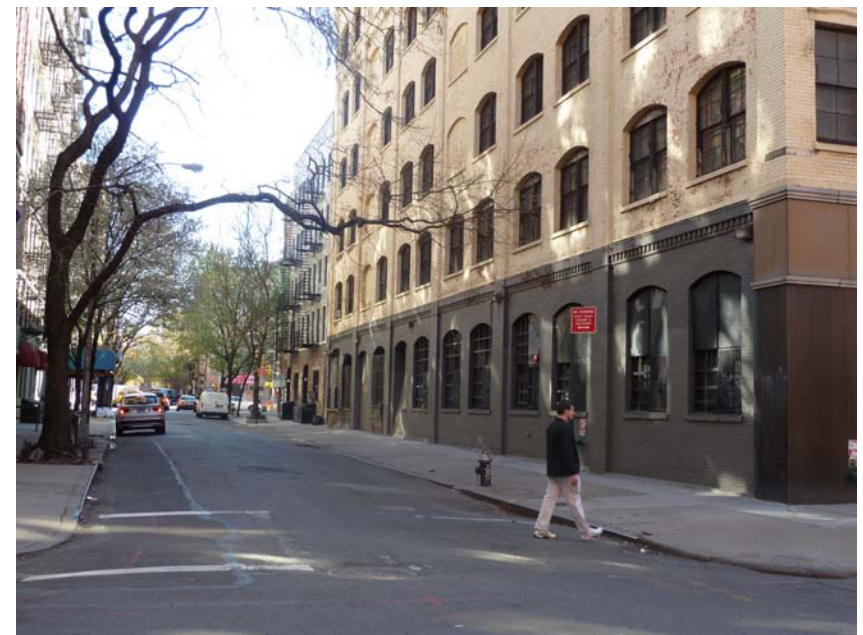
4 Looking south along the Mott St. frontage of the existing building (from Bleeker St.)
