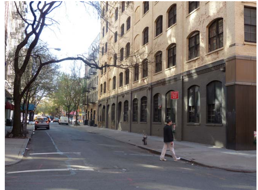
4 Looking south along the Mott St. frontage of the existing building (from Bleecker St.)
