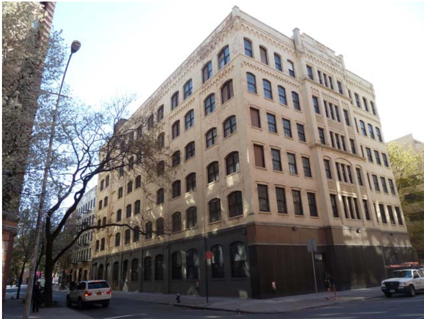
1 Existing building on the Project Site (from corner Bleecker St. and Mott St.)
