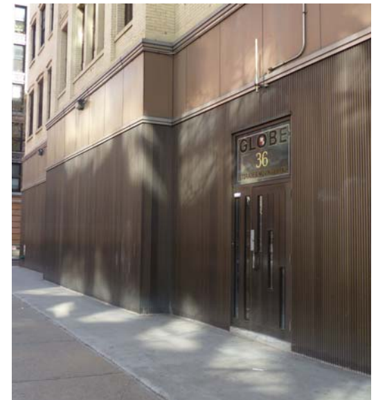
5 Existing facade at Bleeker Street
