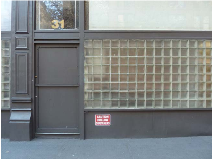
13 Entrance and façade detail (31 Bleeker St.)
