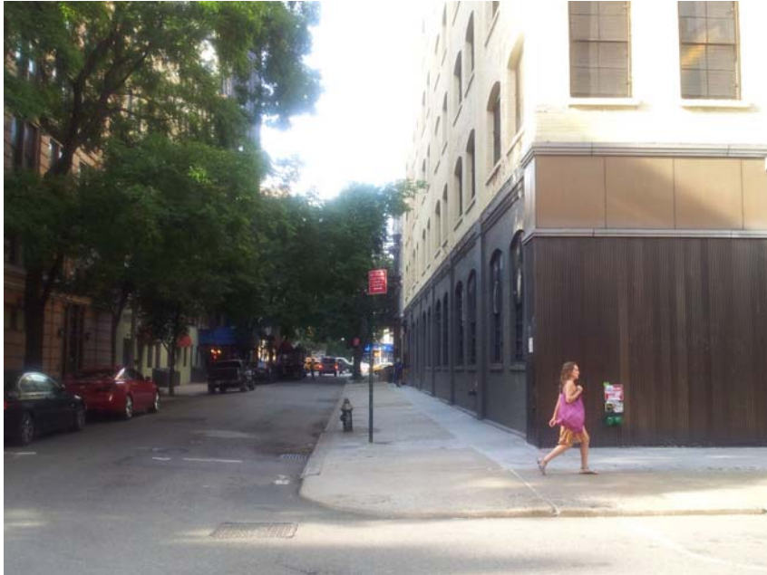
1 Looking south across Bleeker St. along the Mott St. frontage of the building
