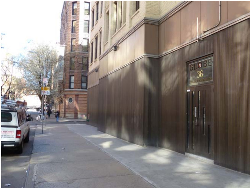
1 Looking east along the Bleecker St. frontage of the building
