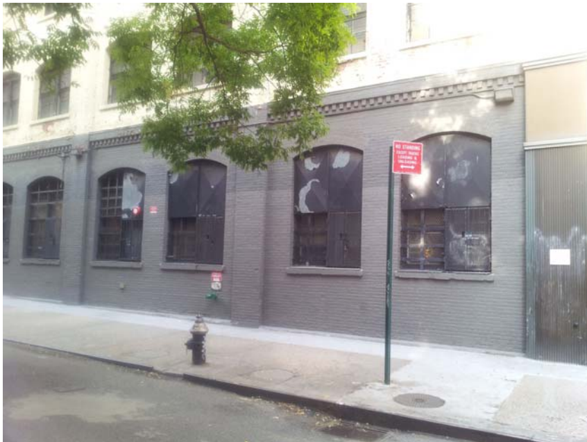
3 Looking southwest across Mott St. from the corner of Bleeker and Mott Sts.
