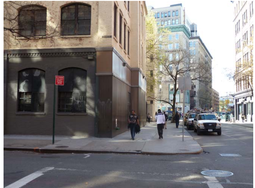
2 Looking west along the Bleecker St. frontage of the building
