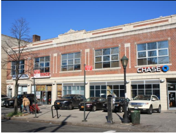
Figure 9- 1: Commercial building with parking on the Eastern Parkway Scenic Landmark
