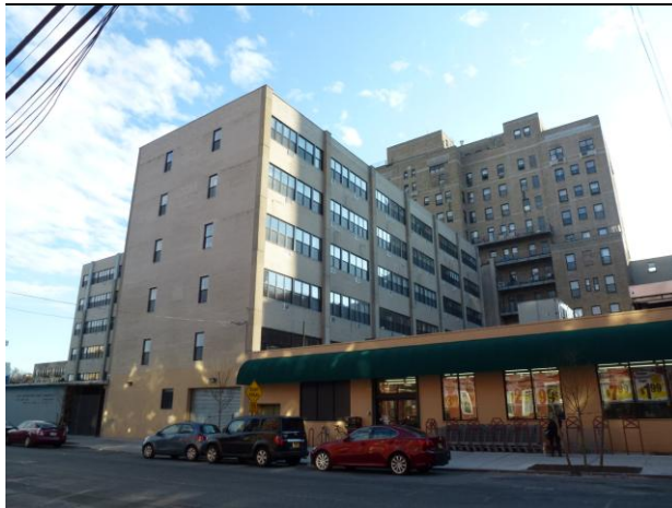
Figure 9- 8: Former Interfaith Hospital complex, looking south from St. Marks Ave.
