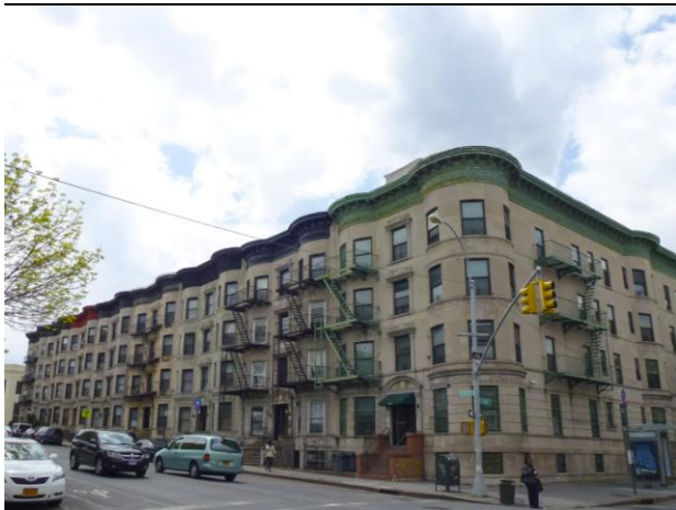
Figure 9- 3: Existing multi-family buildings on the west side of Bedford Avenue
