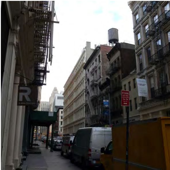
EXISTING VIEW DOWN FRANKLIN, FROM WEST
