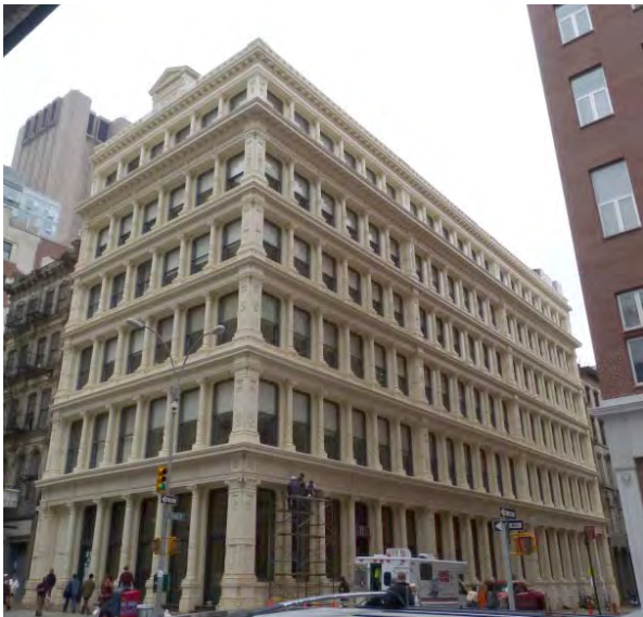
EXISTING VIEW FROM CORNER OF BROADWAY & FRANKLIN
