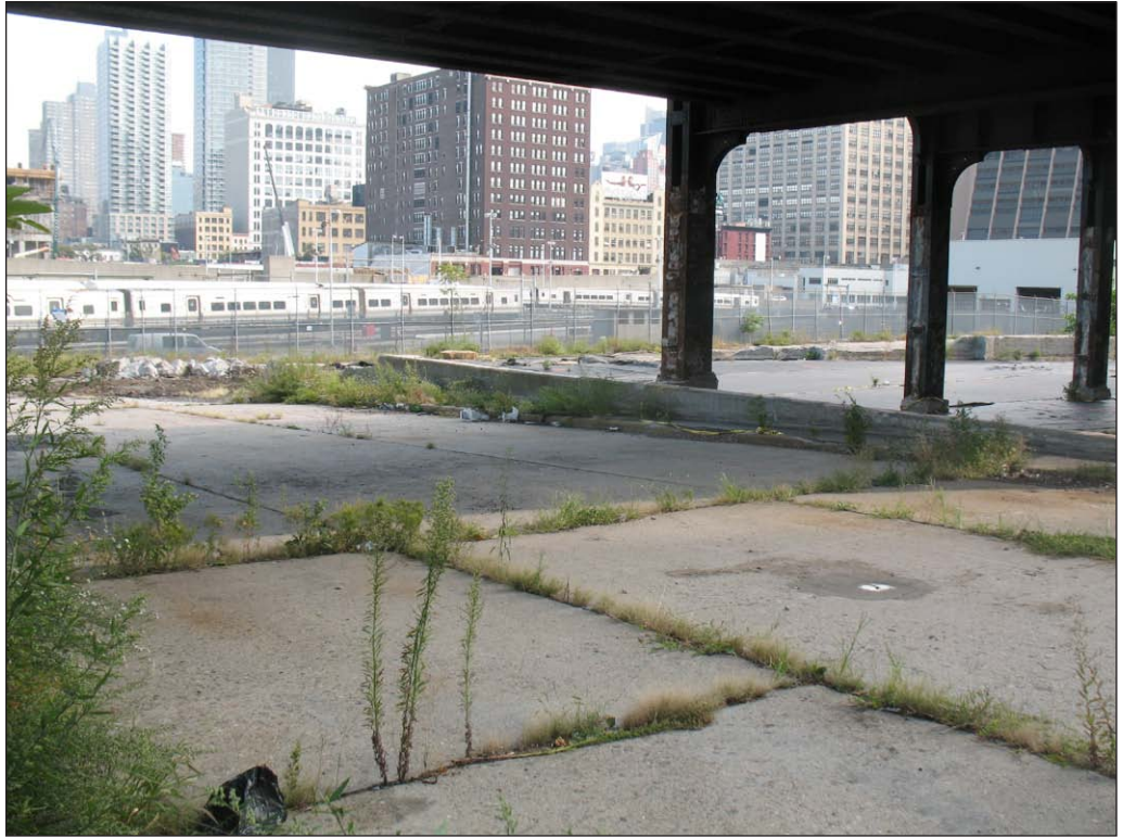
View looking northeast from West 30th Street and Eleventh Avenue 3
