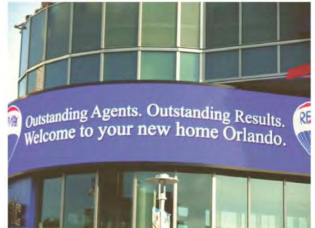
Northeast Corner from W Church St
