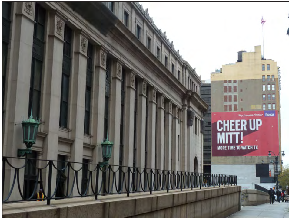
View along West 33rd Street from Eighth Avenue toward Ninth Avenue of existing signage located west of the James A. Farley Building.
