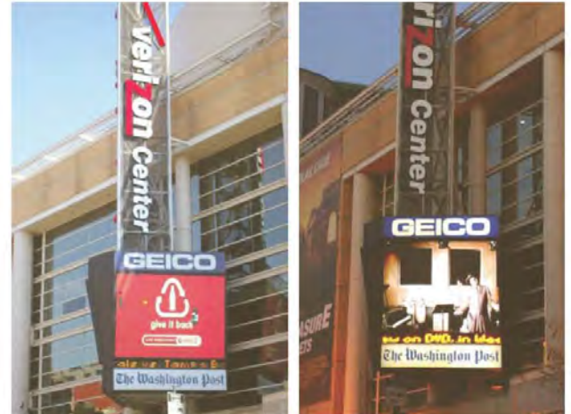
West Facade from South on 7th St NW
