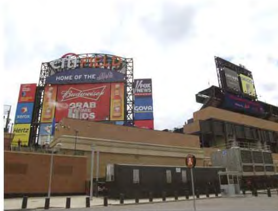
Outfield, North Facade from Parking
