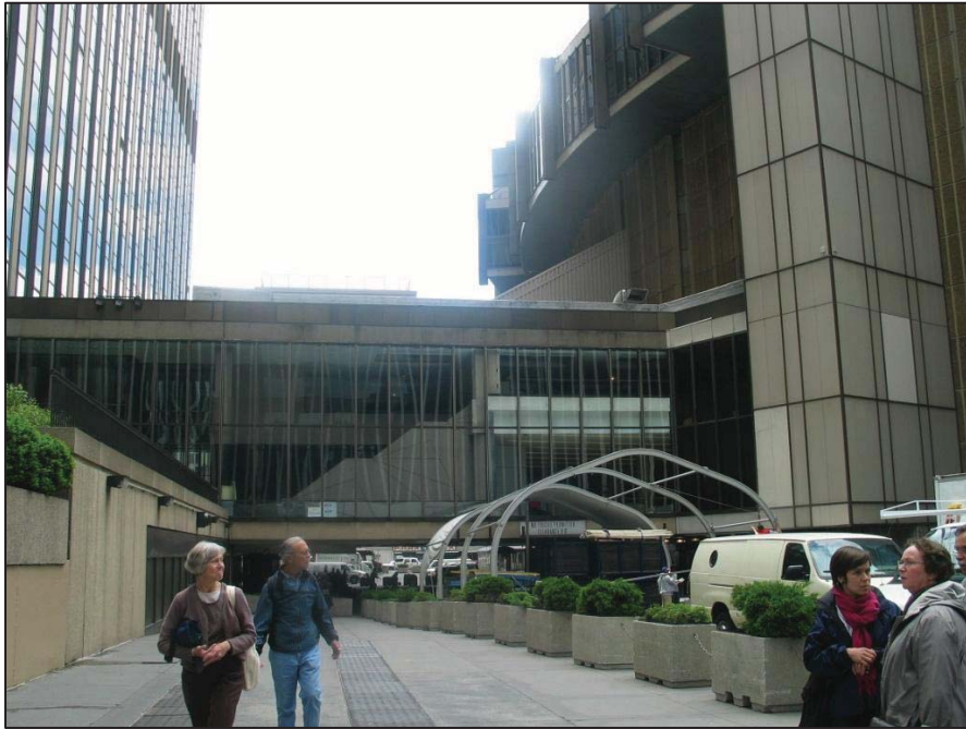
Pedestrian bridge connection the Garden (on the right) with 2 Penn Plaza (on the left). View from midblock pedestrian way along West 33rd Street, looking south.
