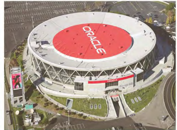
Birds Eye View of South East Facade
