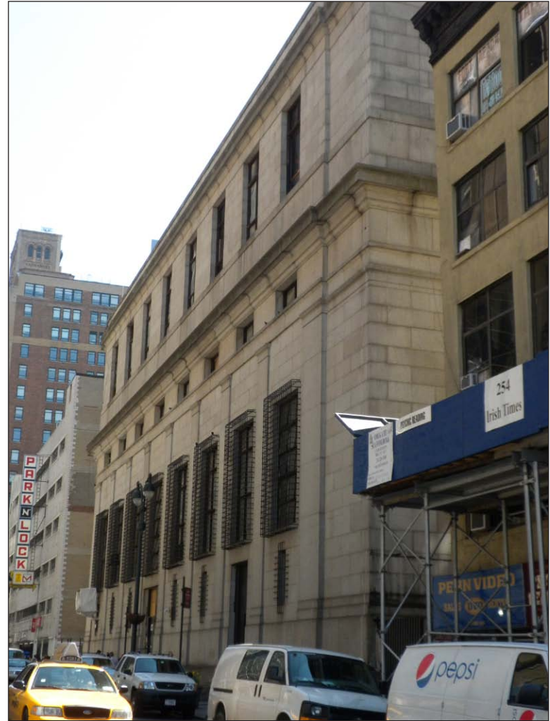
Penn Station Service Building 10
