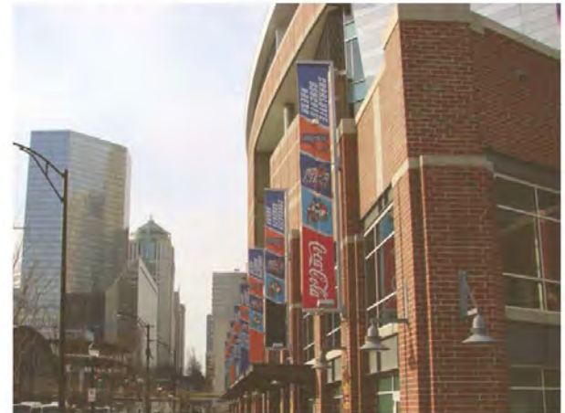
Southwest Facade from E Trade St
