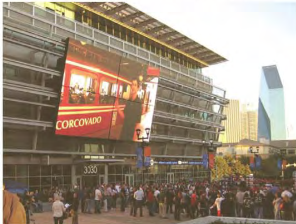
East Plaza Facade facing Southwest from Arena
