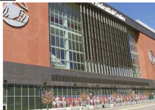
East Facade from Mulberry Street
