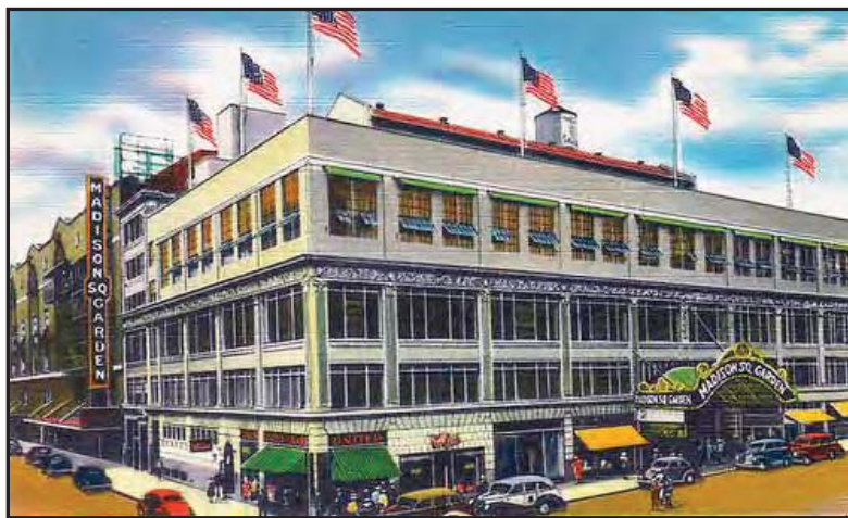
The Garden's facility at Eighth Avenue and 50th Street, constructed in 1925
