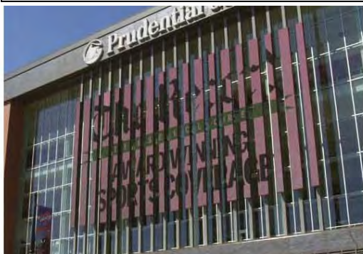
East Facade from Mulberry Street
