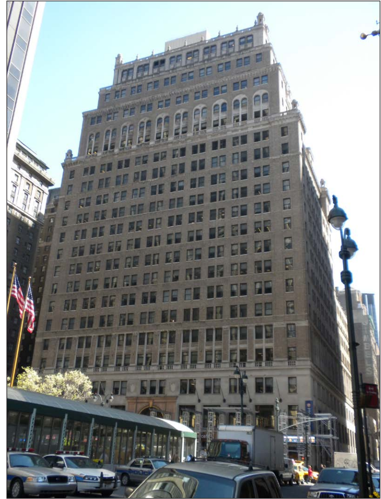
Equitable Life Assurance Company Building 6
