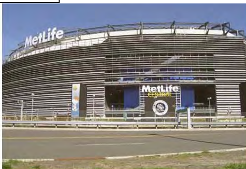
South Facade from Peripheral Rd
