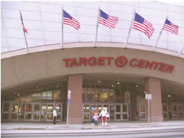
Southeast Facade from N 1st Ave
