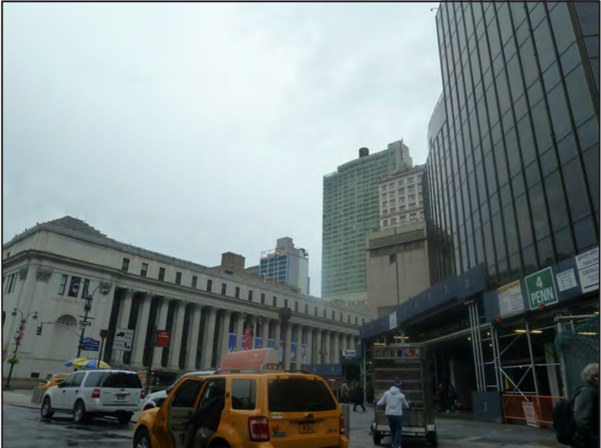
View of the James A. Farley Building from West 31st Street with the Garden in the foreground
