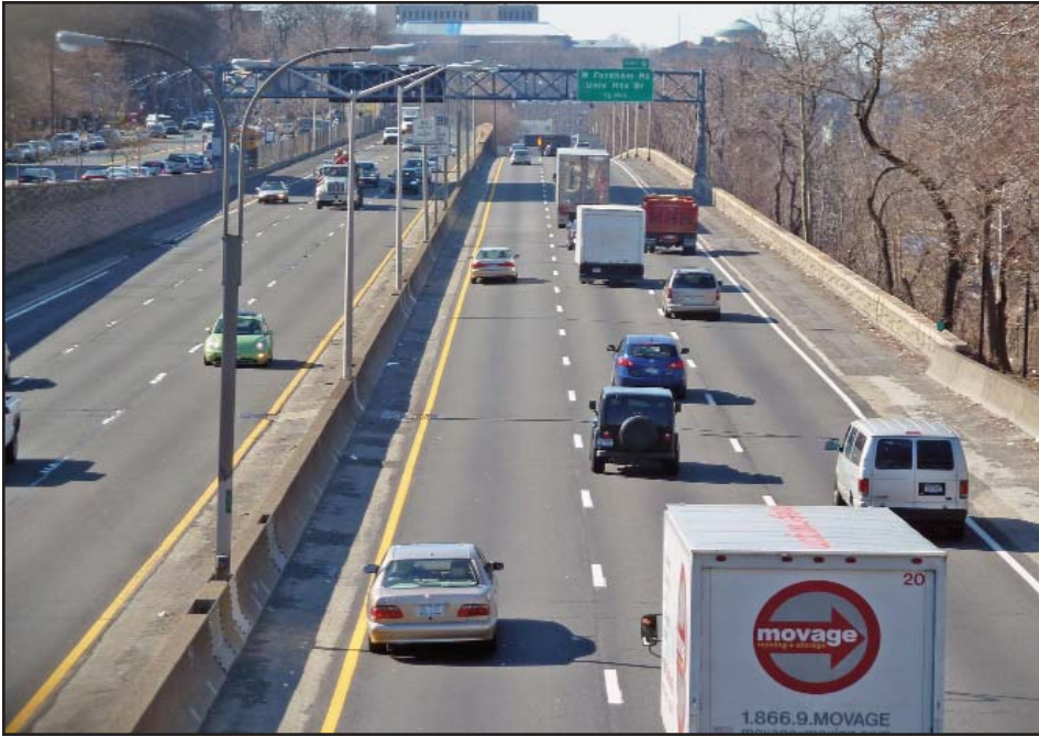
13. View of the Major Deegan Expressway looking south from West 225th St
