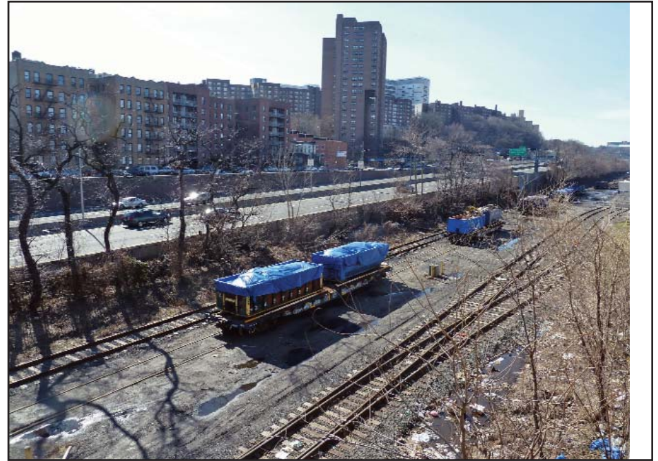
14. View of the Major Deegan Expressway and decommissioned Conrail railroad
