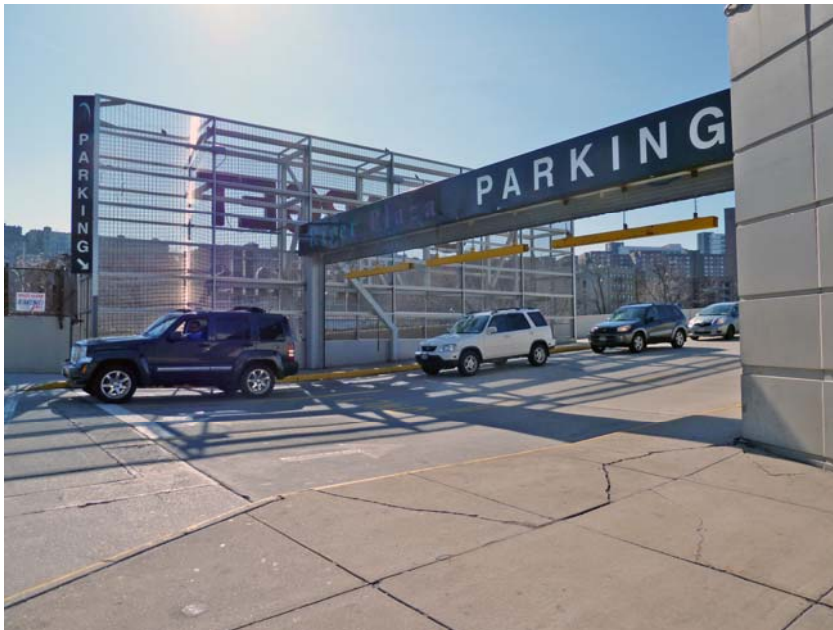
3. View of roof parking entrance/exit at the intersection of W. 225 th St and
