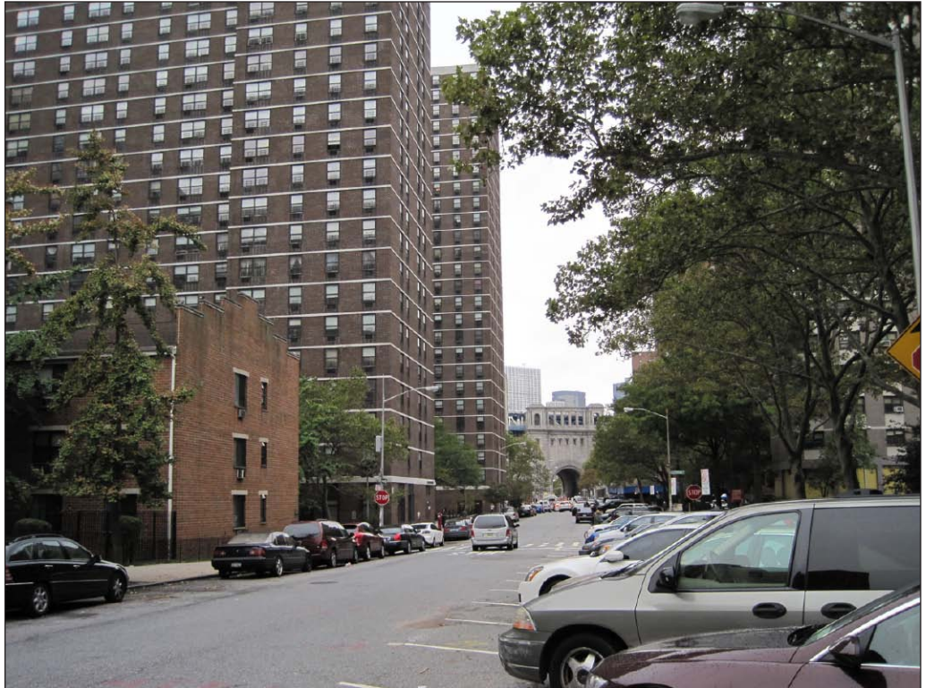
View west on Cherry Street from near Two Bridges Townhouses 21
