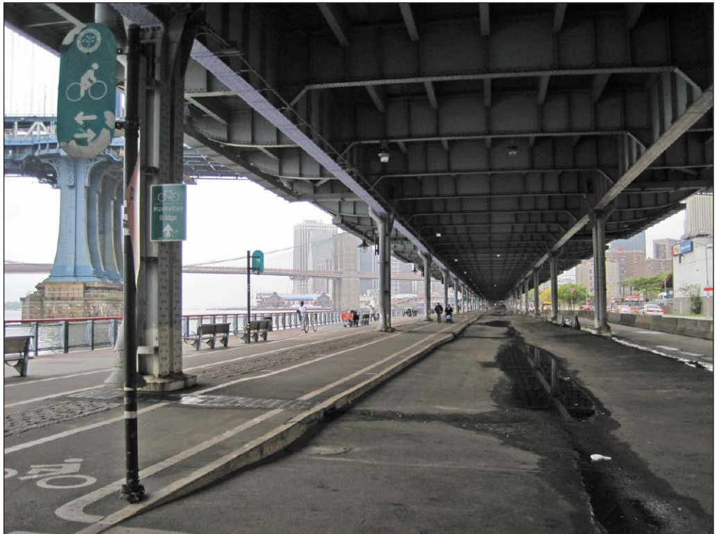
View west under the FDR Drive 11
