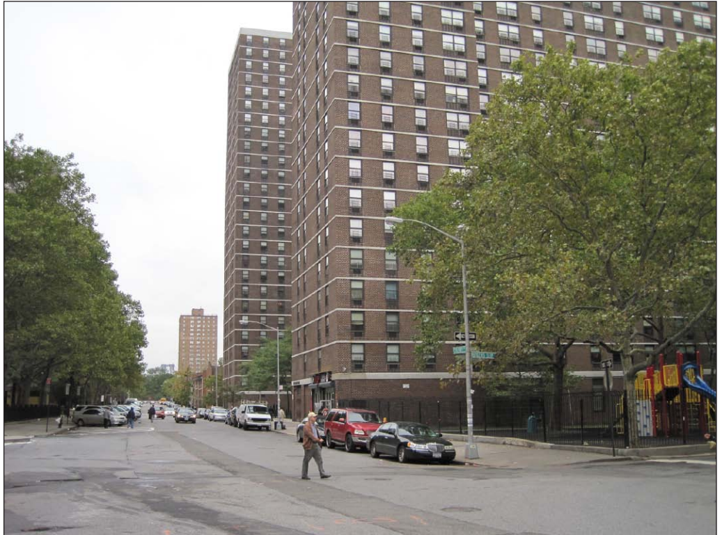
View east on Cherry Street from Rutgers Slip 3
