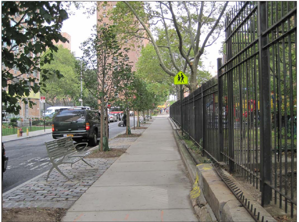
View north on Rutgers Slip from South Street 12
