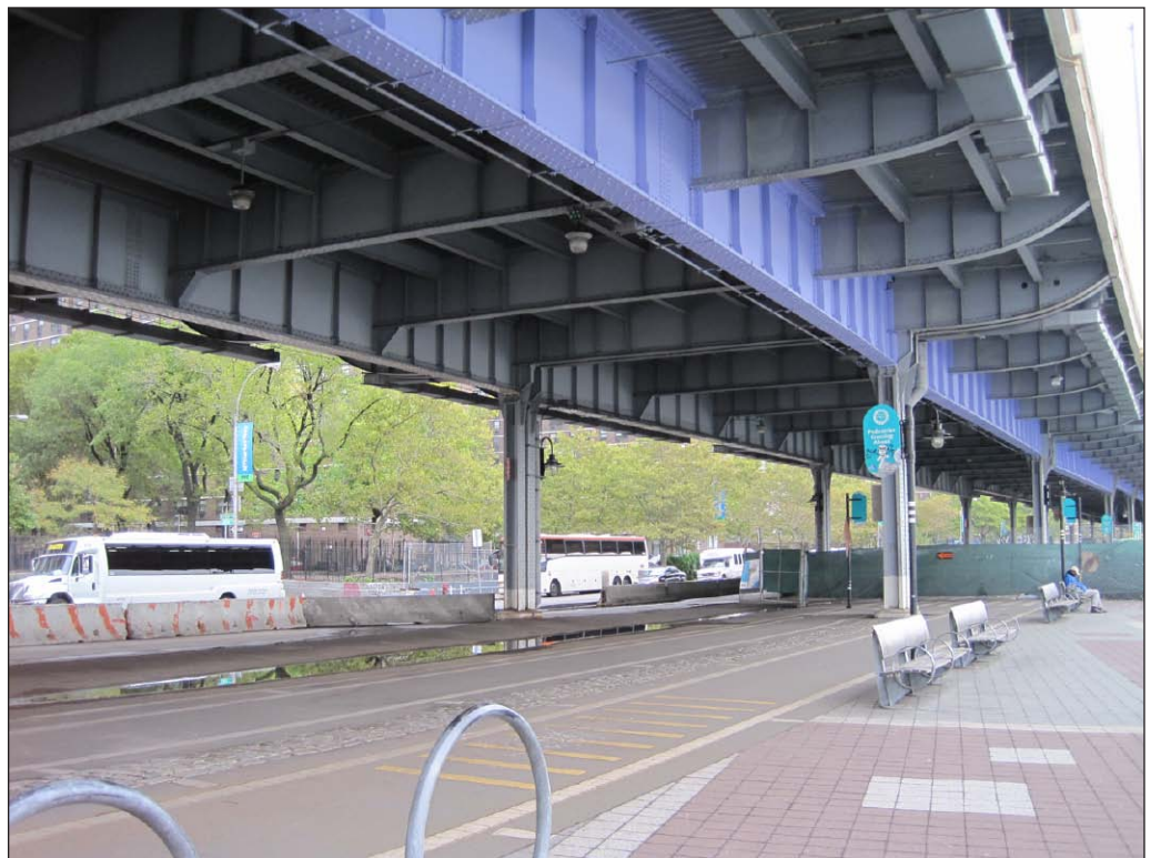
View northeast to project site from esplanade 24
