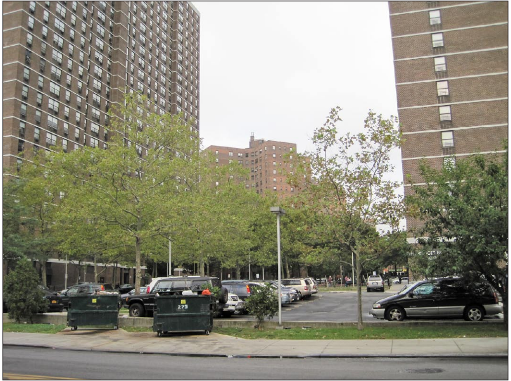
View north from South Street 1
