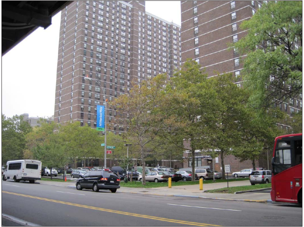
View northwest from South Street at former Jefferson Street 1
