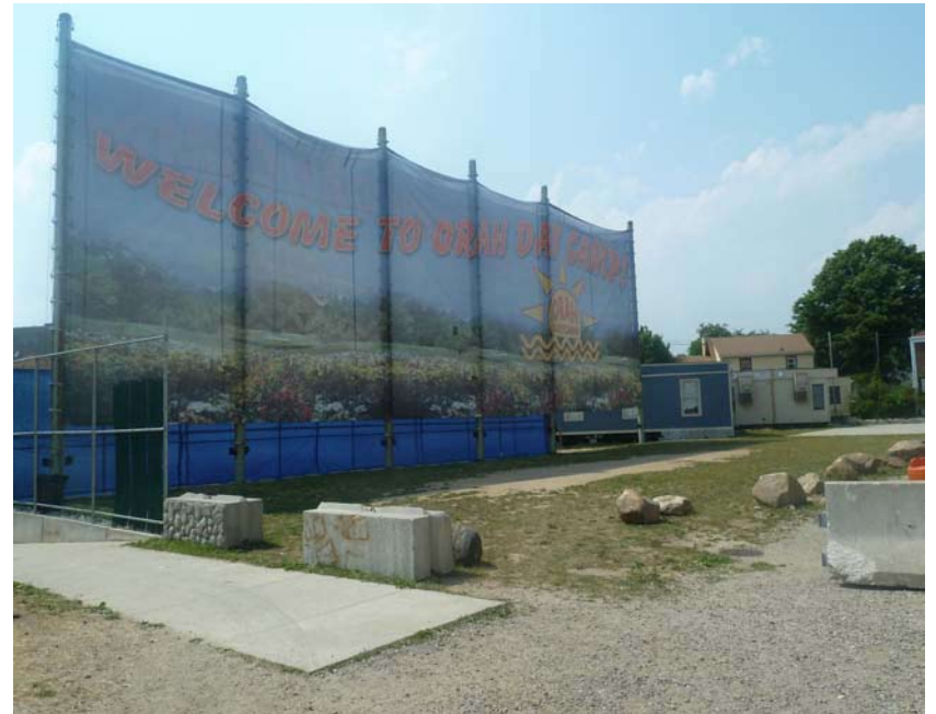
2 Temporary Structures on Beach 12 th Street.
