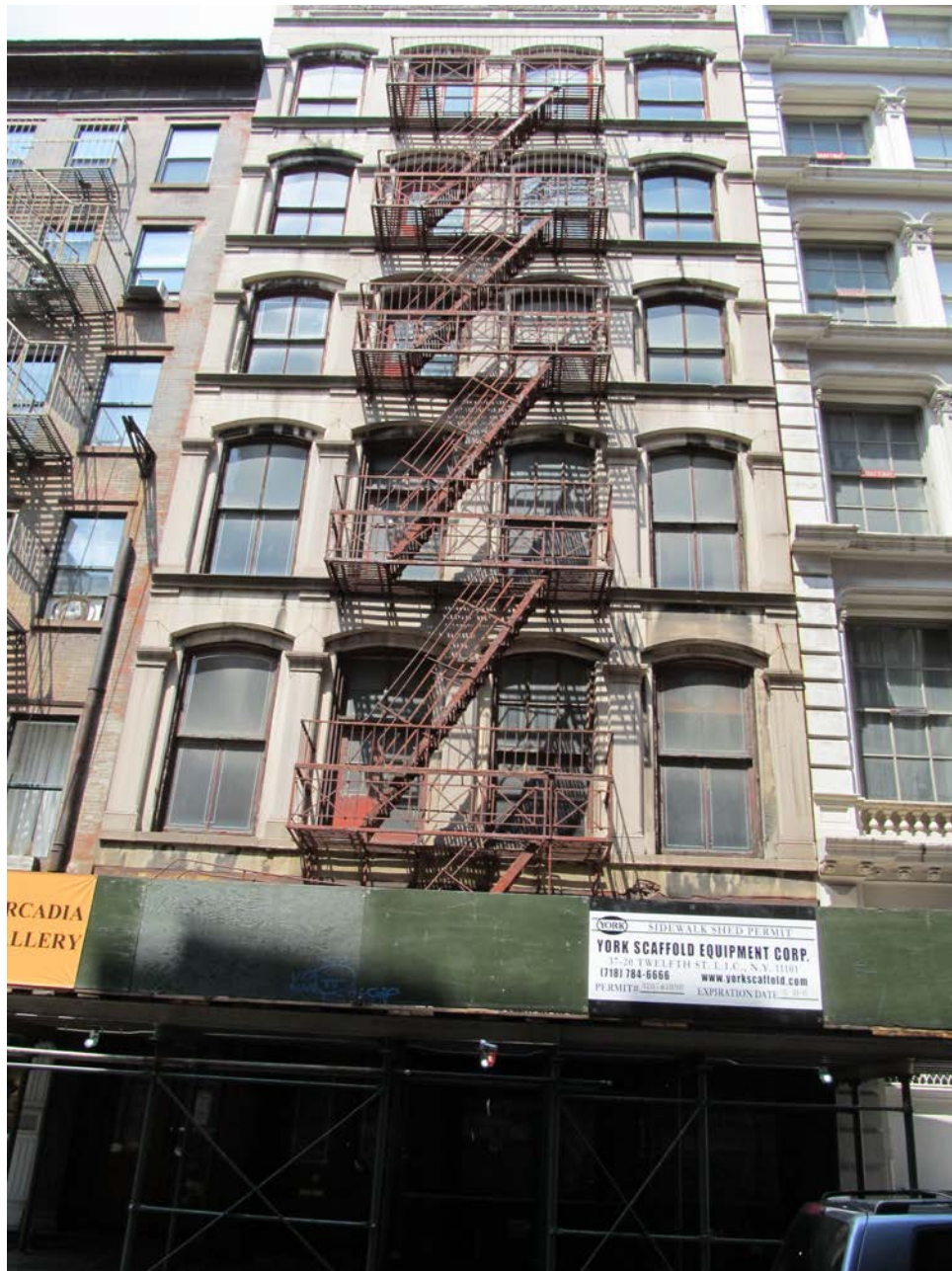
1. Looking at the project building from Greene Street
