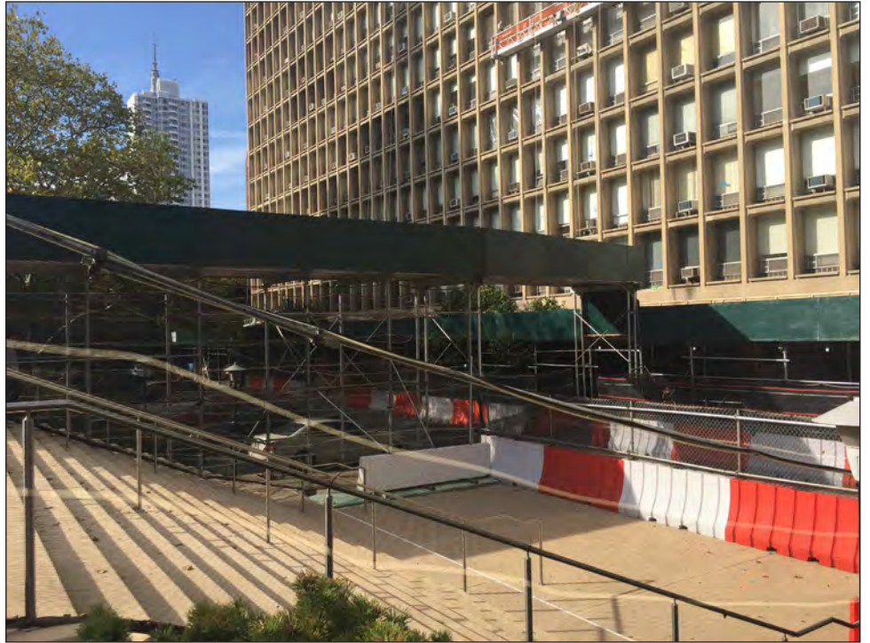
View Northwest of South Parking Lot 3
