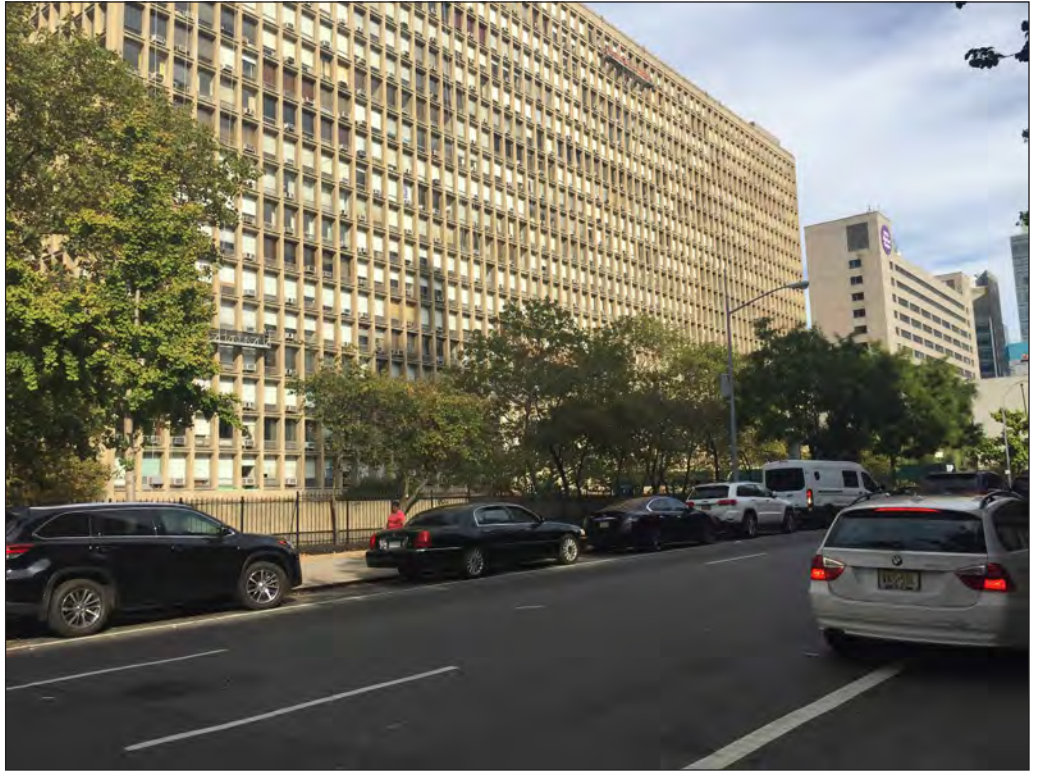
View North from E. 30th Street 1
