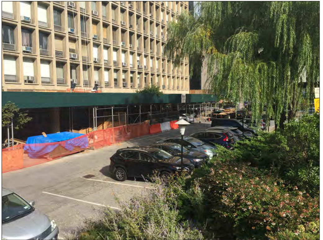
View Northeast of South Parking Lot 2
