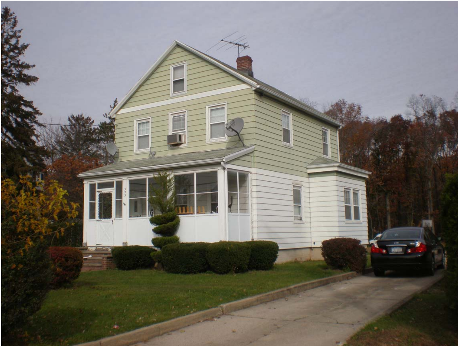
Photograph 3. Front view of a residential dwelling on 323 Arden Ave to be demolished
