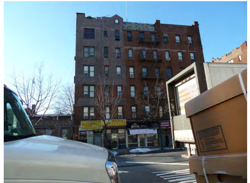
4 View of the 6-story building on Block 1324, Lots 18 and 35.
