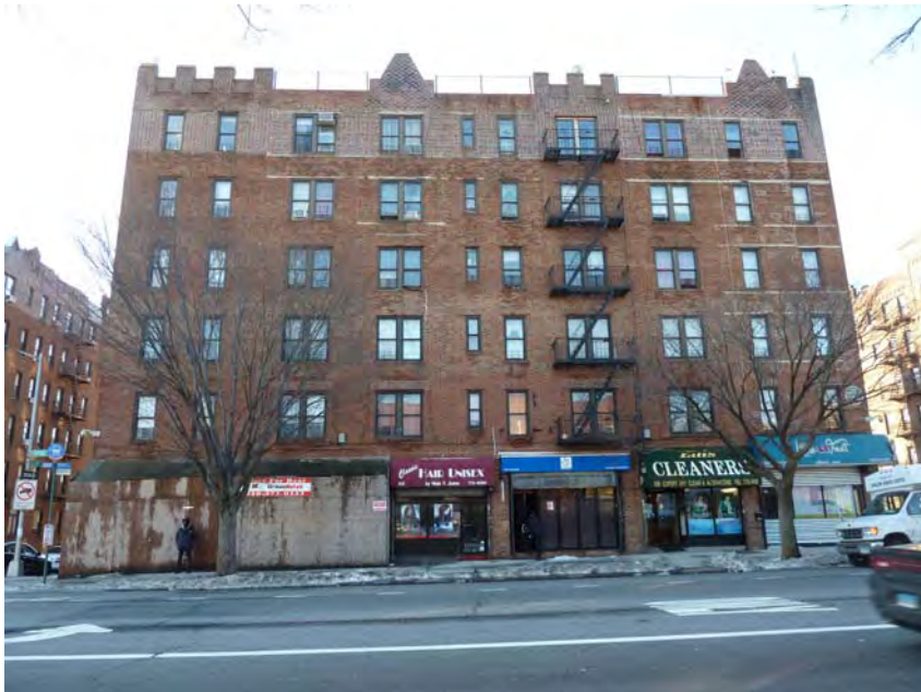
3 View of the 6-story building on Block 1323, Lot 17
