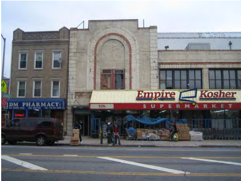
1 View north across Empire Blvd. towards the 2- and 3-story buildings on the project site (located on Lots 74 and 66, respectively).
