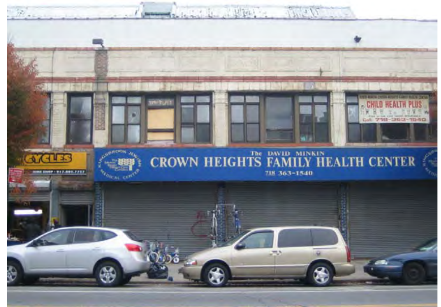
2 View north across Empire Blvd. towards the 2-story building on the project Site (located on Lot 66).
