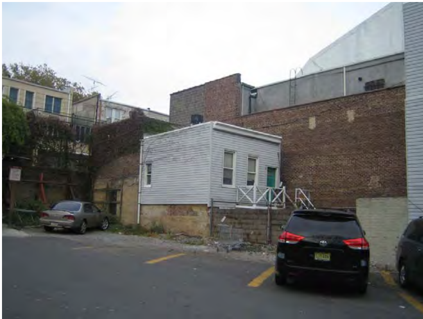
3 View of the 2-story former residential building (vacant) in the rear of Lot 74.
