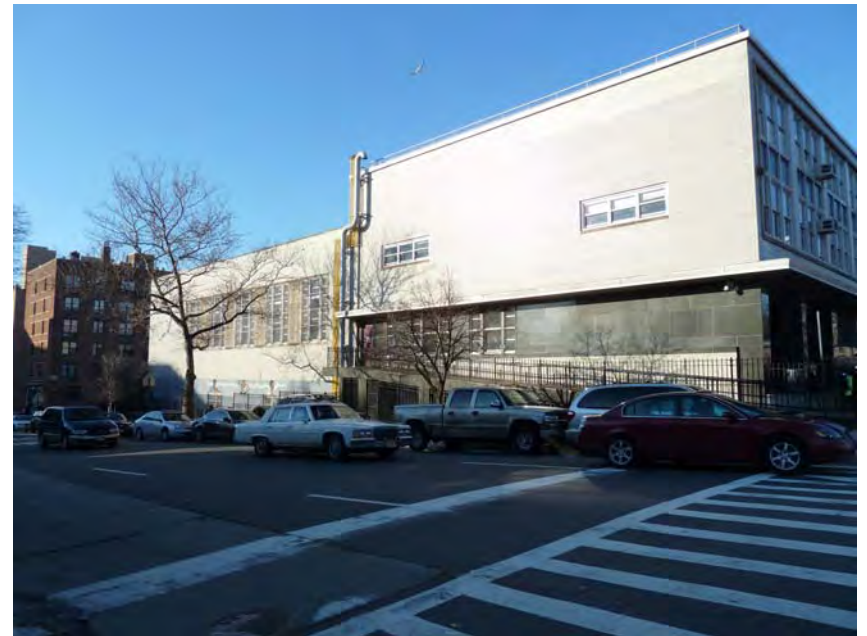
4 View southeast across New York Ave. towards Brooklyn M.S. 61
