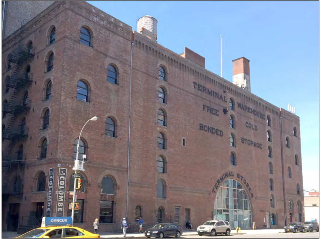
West Chelsea Historic District (S/NR-eligible, NYCL)—Northwest view to the New York Terminal Warehouse Company's Central Stores Complex
