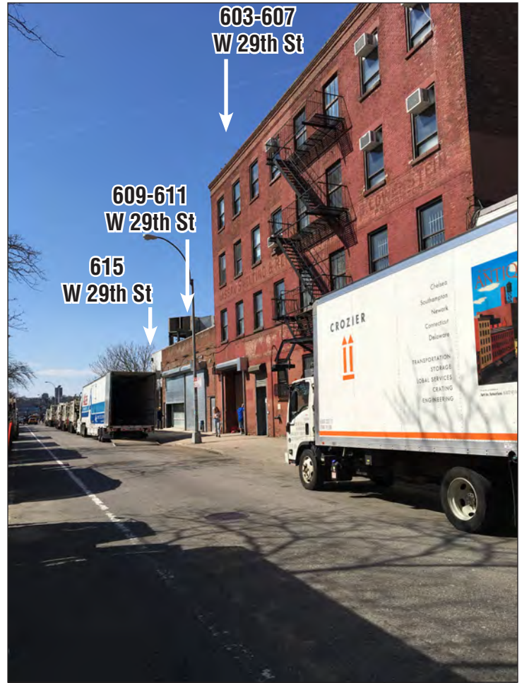
Northwest view of the four-story warehouse and garage on Lot 12 1
