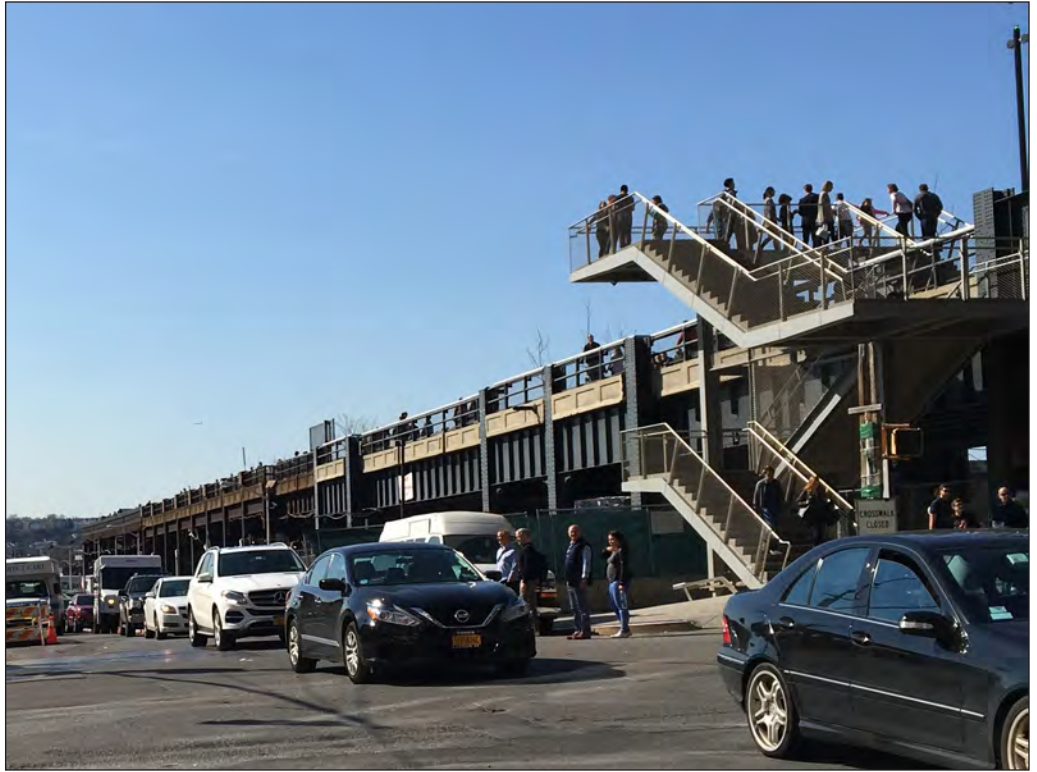
The High Line (S/NR-eligible) 5 Northwest view from Eleventh Avenue and West 30th Street
