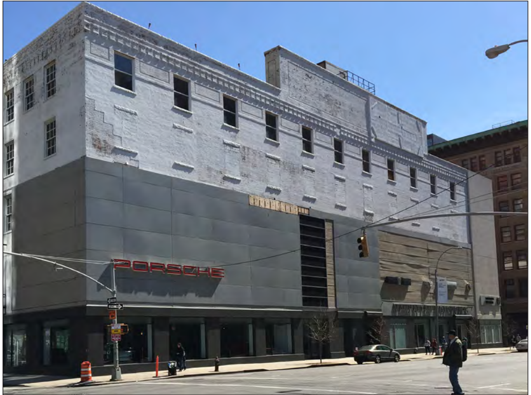
West Chelsea Historic District (S/NR-eligible, NYCL)—Southeast view from West 28th Street and Eleventh Avenue
