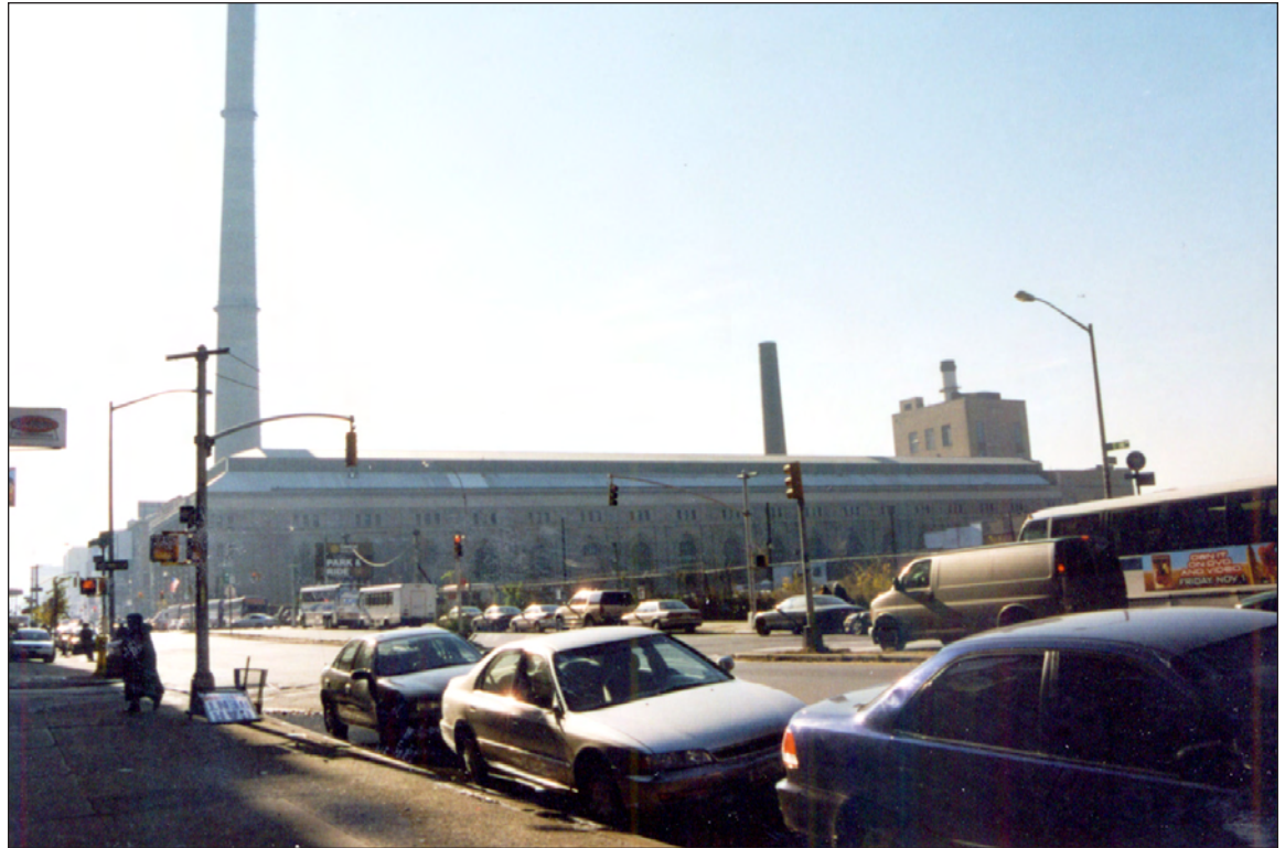
View south of the Con Edison Power House, as seen from West End Avenue 13
