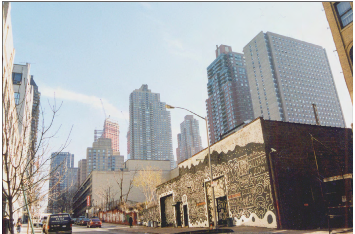
View southeast of the project site along West 61st Street 2
