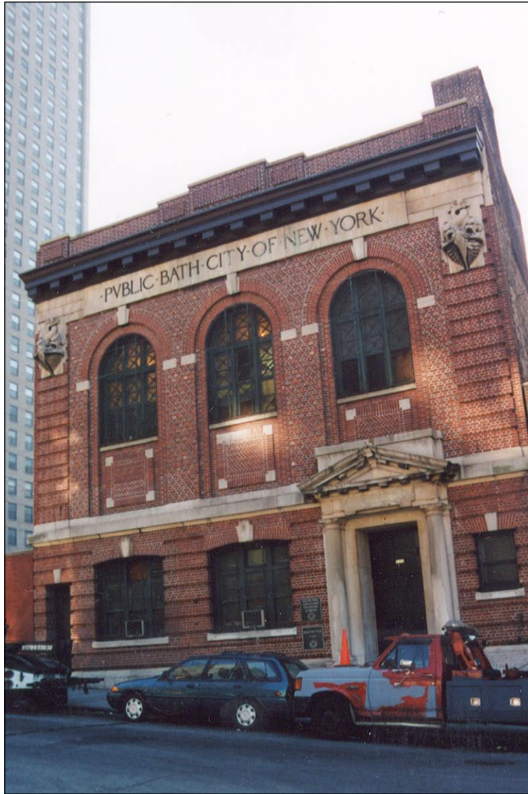
View south of the West 60th Street Public Bath facade 3
