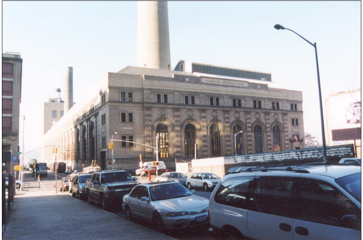
View northwest of the Consolidated Edison Power House 5
