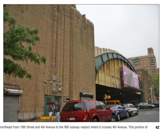
Looking northeast from 10th Street and 4th Avenue to the IND subway viaduct where it crosses 4th Avenue. This portion of the viaduct, consisting of a steel-arch and brick piers designed in the Art Deco-style, houses the 4th Avenue subway station, which is listed on the S/NR
