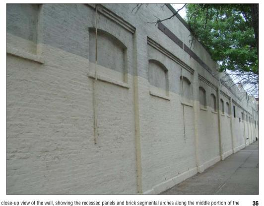
A close-up view of the wall, showing the recessed panels and brick segmental arches along the middle portion of the structure along 3rd Avenue
