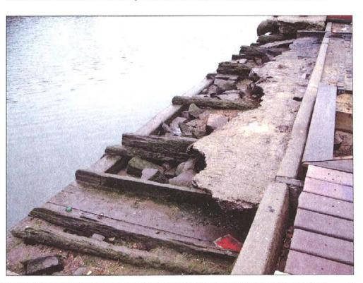
A view of the deteriorating bulkhead at the terminus of 2nd Street on the west side of the Gowanus Canal.
