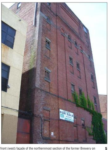
The front (west) façade of the northernmost section of the former Brewery on Bond Street at 4th Street. The tall brickstructure has a both round-arch and rectangular windows, and an ornamental brick cornice
