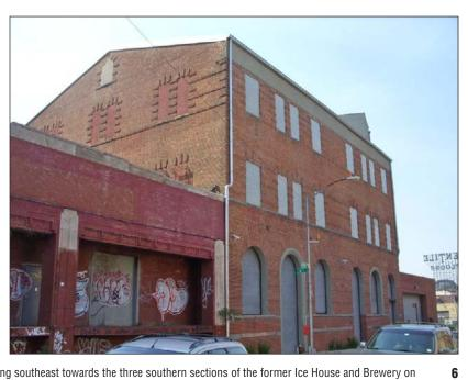
Looking southeast towards the three southern sections of the former Ice House and Brewery on Bond Street. The peak-roofed section (center), which was round-arched windows and projecting brickwork suggesting quoins and voussoirs, is the earliest section, built ca. 1900
