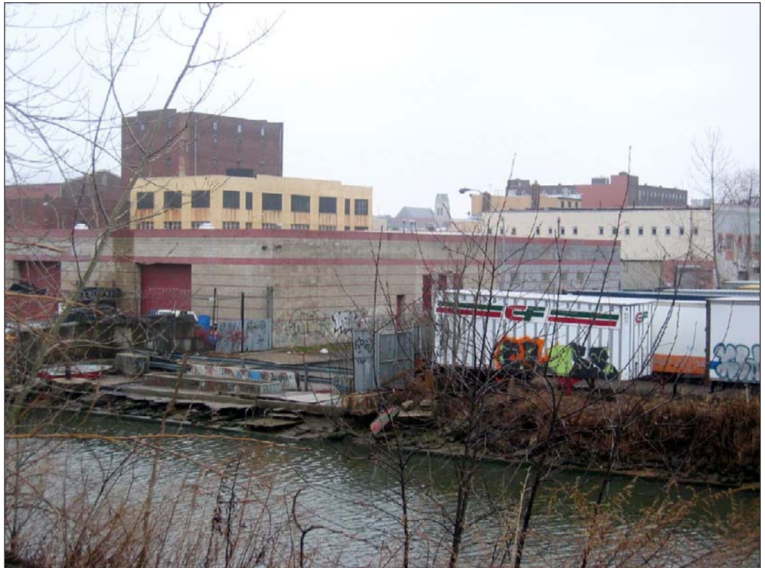
Facing west towards project site (end of Second Street) from east side of Gowanus Canal 10
