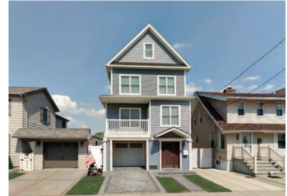
Example of new single-family flood resilient construction in Hamilton Beach, Queens.
