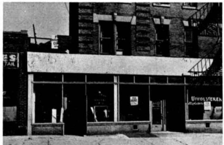
Excessive development of retail frontage results in vacancy. Melrose section of The Bronx.
