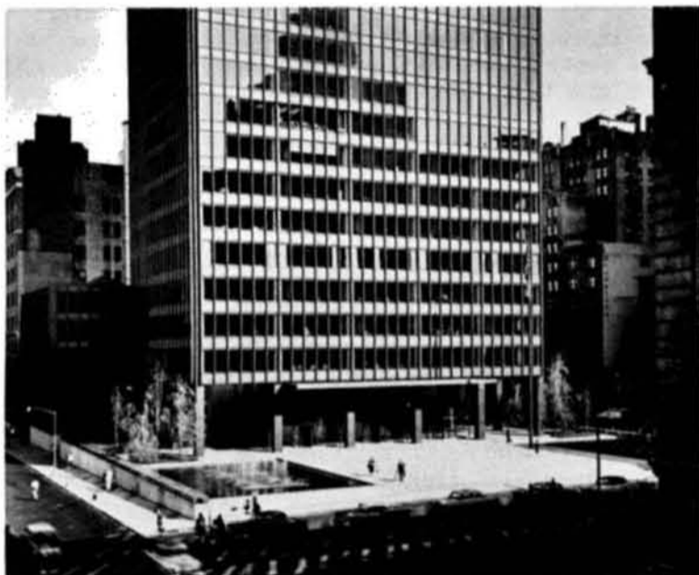
Open area at ground level permits a higher rise before a setback is required, as well as a bonus in Floor Area Ratio. Seagram Building, Manhattan.
