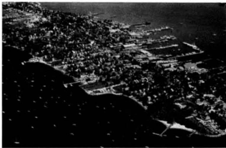
Boat docking and servicing facilities at City Island, Bronx.
