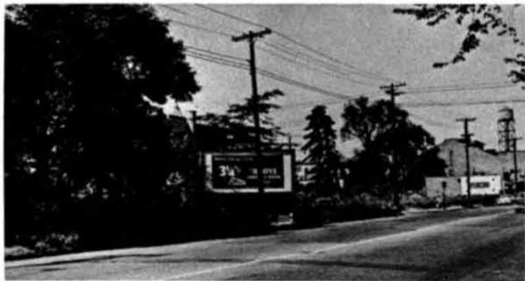
Excessive strip zoning for commercial use results in no use at all. East Bronx.
