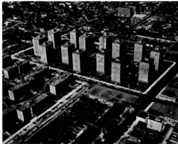
Example of good spacing in large-scale development such as would be encouraged by minimum spacing formula. Queensview, Queens.
