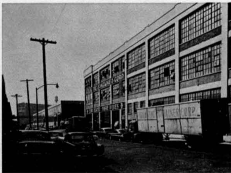
Inadequate off-street parking and loading facilities result in parking on sidewalk area.
