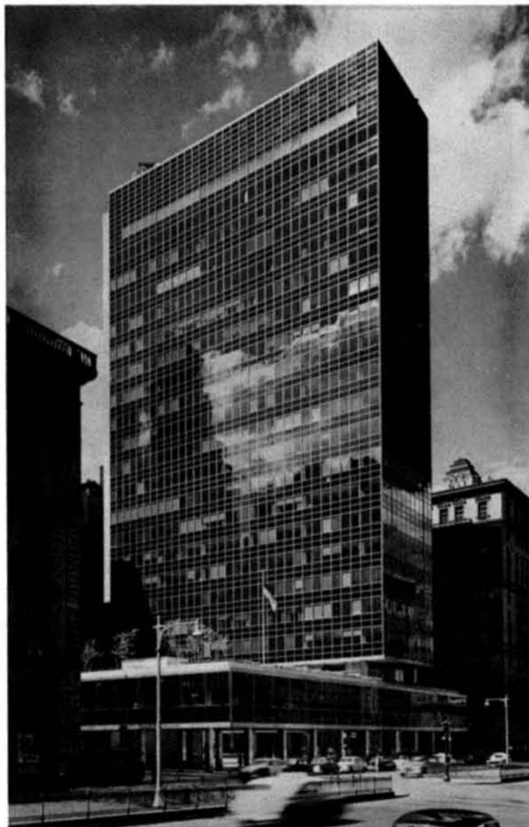
Tower covering less than 40% of the lot area may pierce sky exposure plane. Lever House, Manhattan.
