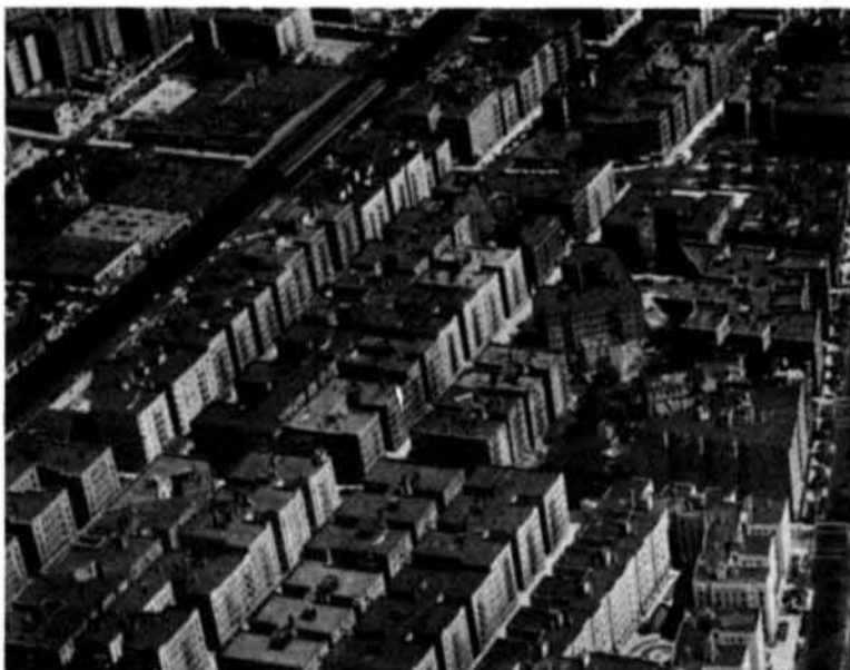
Most of these buildings have inadequate light, air, and open space.
