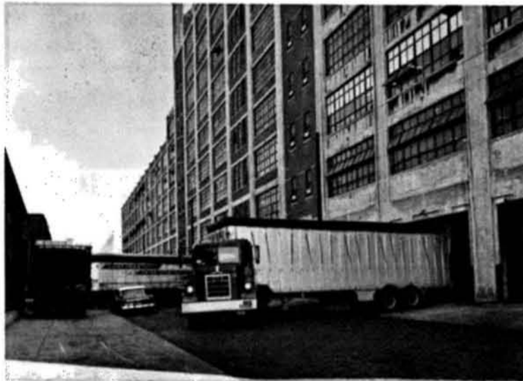
Inadequate off-street loading facilities result in blockage of street and sidewalk.
