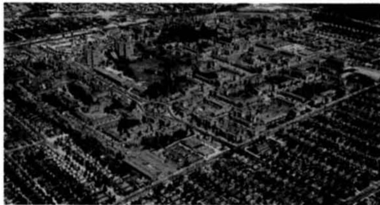
Example of good large-scale residential development, including well-located shopping centers. Fresh Meadows, Queens.
