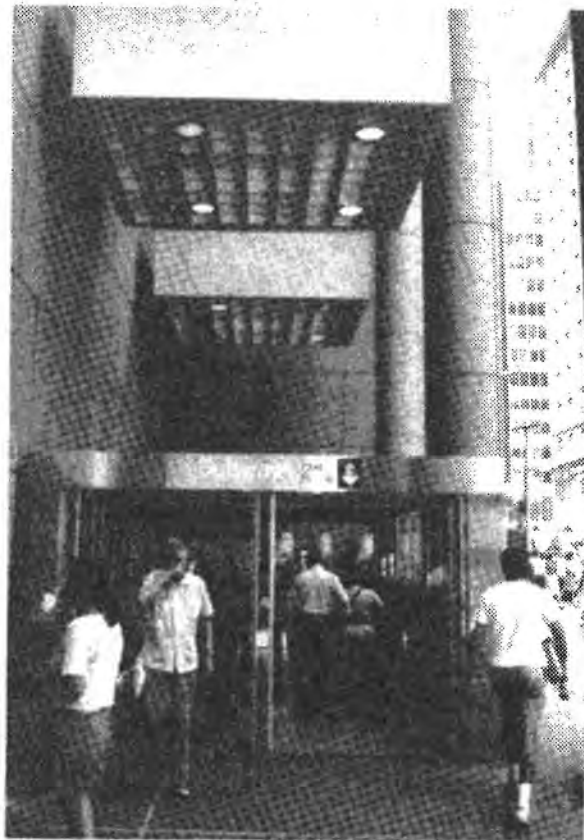
Figure 25. Subway Entrance at Philip Morris.
