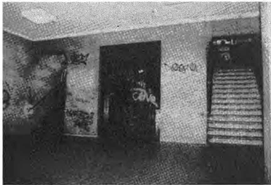
Figure 19. A Neglected Passageway Beneath Pershing Square
