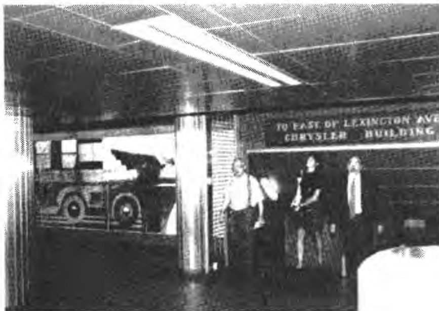
Figure 20. New Finishes in the Grand Central Subway Station
