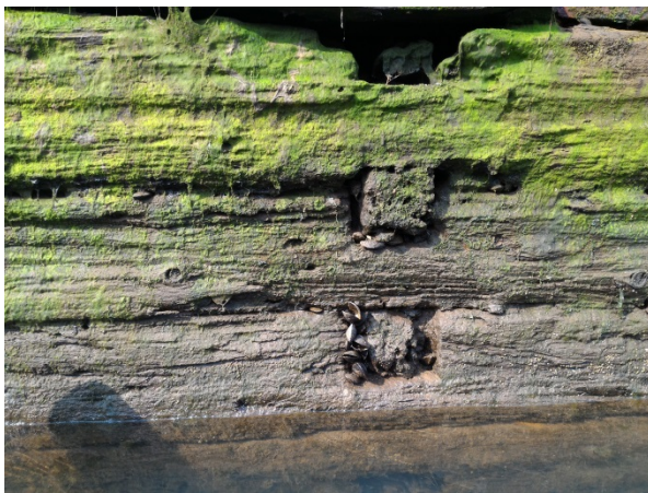
FIGURE 3-4 Mussel Colonization of Degraded Wooden Bulkhead
