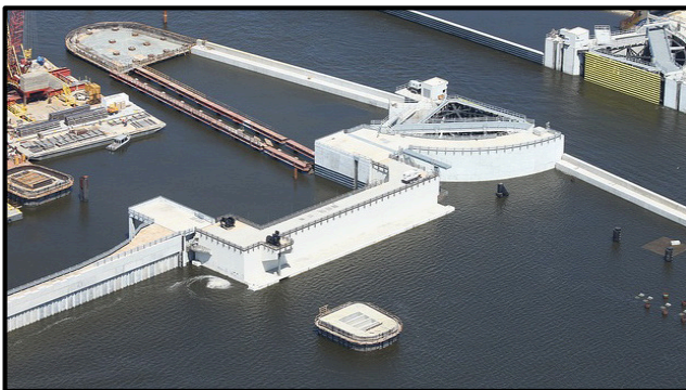
Horizontal sector gates in normal open position recessed into areas adjacent to the channel and clear of navigation. Source: USACE, 2012
