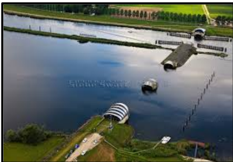
Rubber dams in deflated open position.
