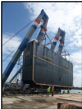
Sliding caisson gate post refurbishment being lowered into normal open position. Source: Becketttrankine.
