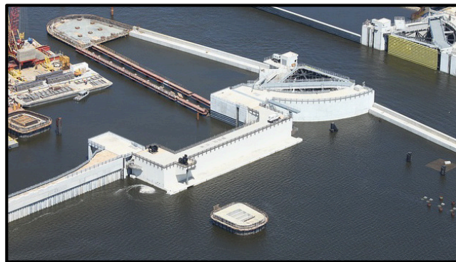
Barge gate in normally closed position on left alongside horizontal rotating sector gates. Source: USACE, 2012
