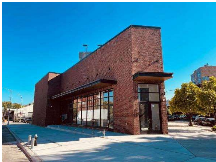
New restaurant space at 113 Hamilton Avenue
