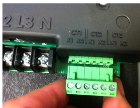
CT Terminal Block Removed
