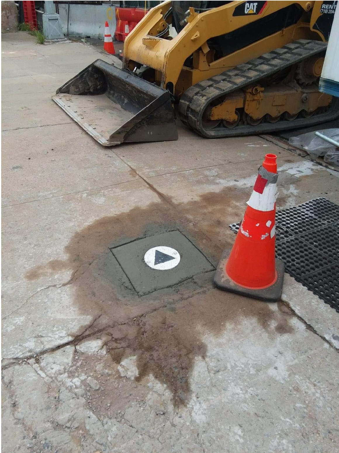
Photo 2: MW-02 manhole replaced and restored
