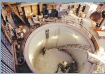
The City's Department of Environmental Protection completed the restoration of the Gowanus Canal's "flushing tunnel," in April 1999. The tunnel conveys fresh water from Buttermilk Channel into the head of Gowanus Canal. In 1992, DEP began designing the repair and restoration of the flushing tunnel and construction began in 1995. The pump (above right) brings harbor water to the Canal at an average rate of 200 million gallons a day.
